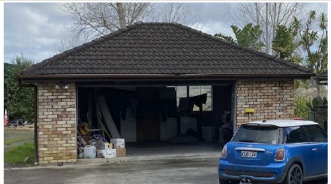
Photograph 10. View of the garage, facing south.
