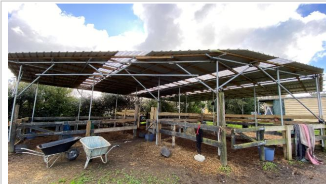
Photograph 13. View of the covered yards, facing northeast.
