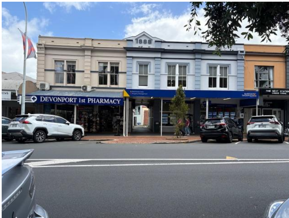
Figure 3-2: Existing Access on Victoria Street
