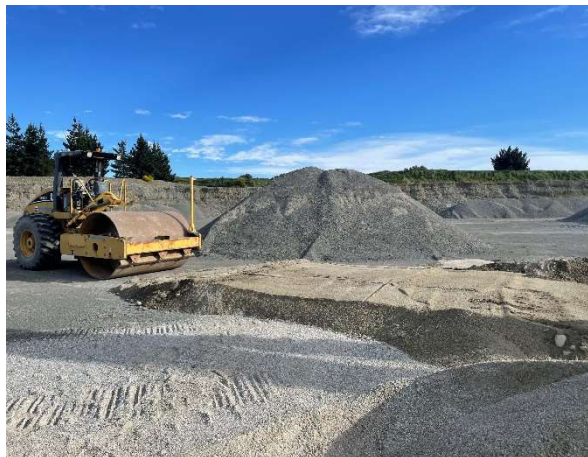
Photograph 5: Trial pad 1 prior to compaction.
