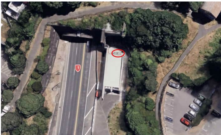
Figure 44 Electrical transformers at the Terrace Tunnel southern portal (image from NZTA)
