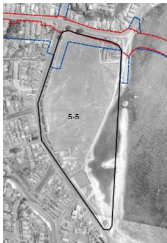
Figure 38 Feature 5-5 (1938) showing in progress land reclamation in the southeast of Kilbirnie Park
