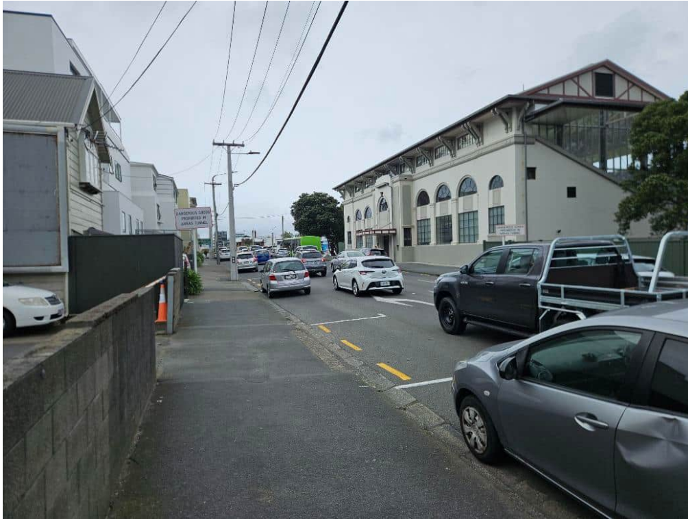
Photo 43: Section 3 General view of Sussex Street, facing north 20-10-2025
