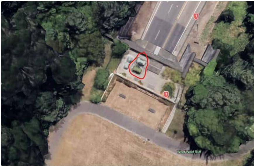
Figure 43 Electrical transformers at the Terrace Tunnel northern portal (image from NZTA)
