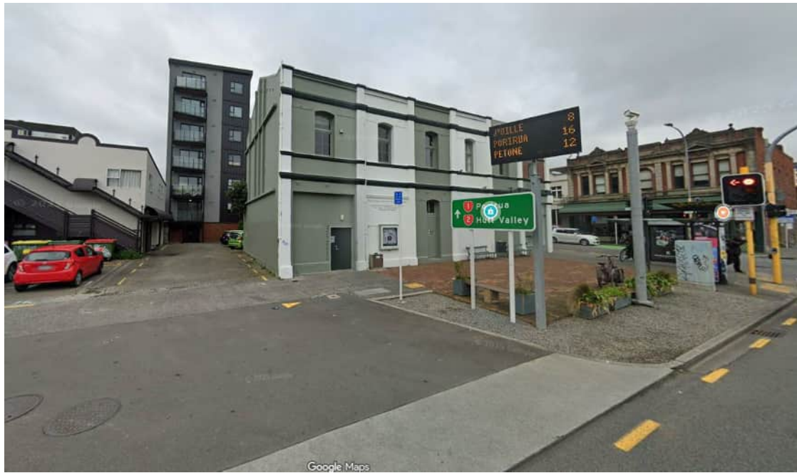
Photo 66: Section 2 Corner of Karo Drive and Cuba Street, facing southwest 10-05-2026
