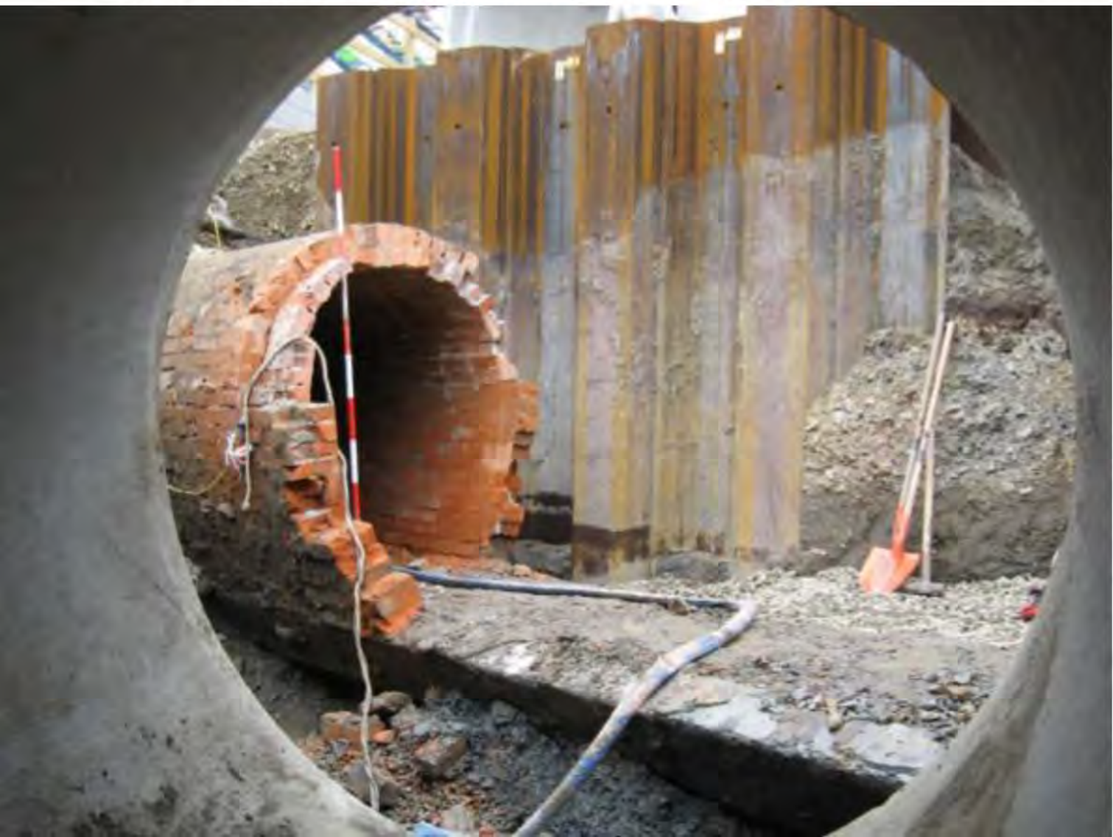
Historic Waimapihi brick culvert uncovered during the Z Energy Vivian Street re-build
