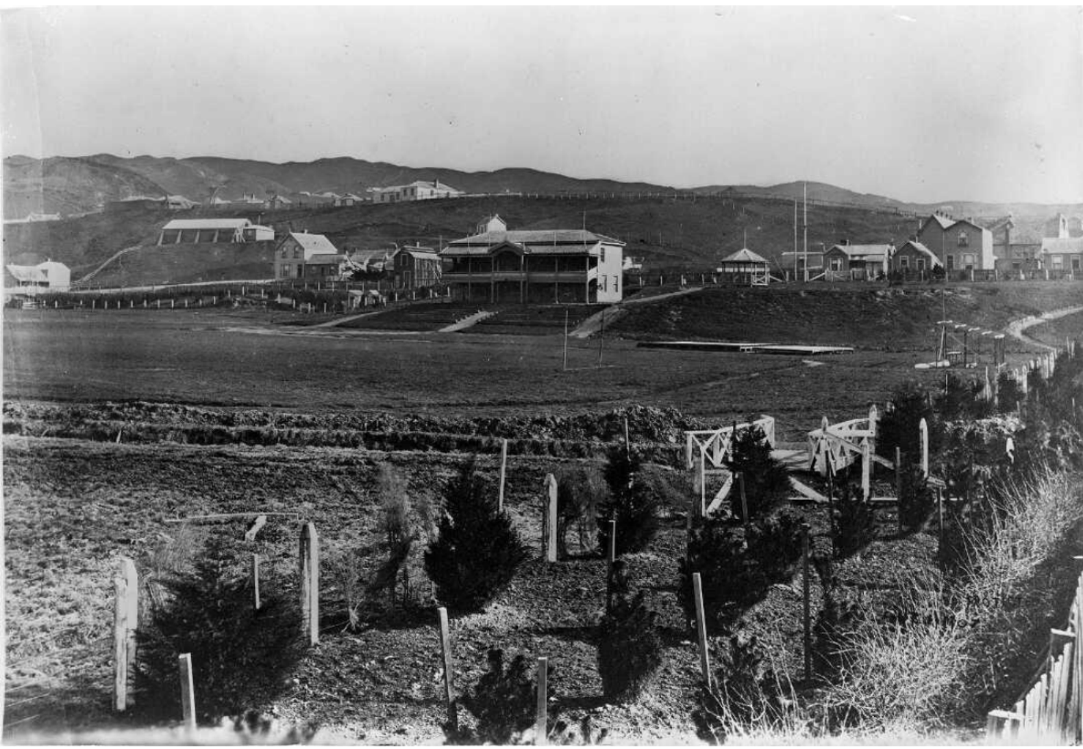
The Basin Reserve 1877 with the Waitangi Stream contained in the drainage ditches in the middle of the photo
