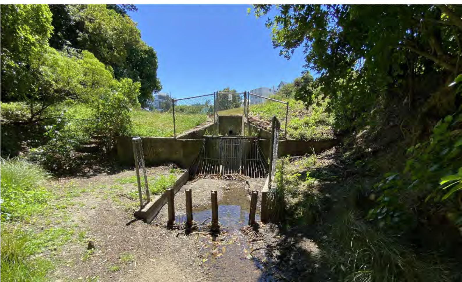
Kumutoto Awa culvert where it drops approximately 11m before being piped under the Terrace Tunnel and motorway
