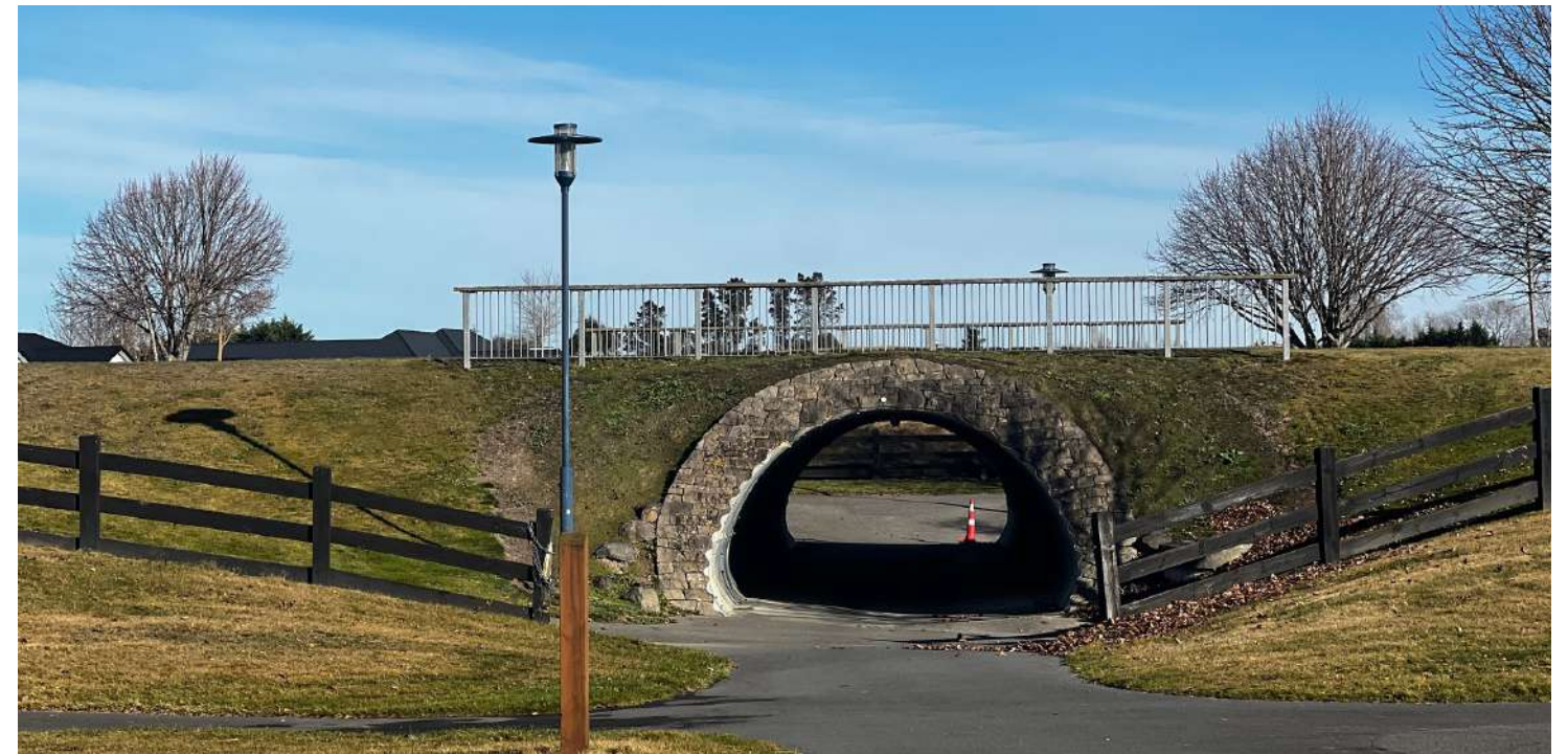
Underpass: This image is taken from north of Pegasus Boulevard, showing pedestrian underpass facilitating movement between north and south of Pegasus Boulevard. There are two underpasses of the same nature within 500m
