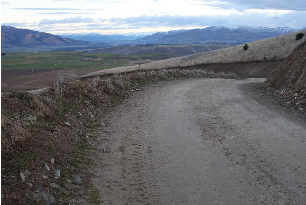
Figure 18: Existing Thomson Gore Road – Edge protection on modified sections
