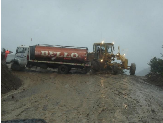
Figure 14: Overseas example of silt rich surfacing in winter months
