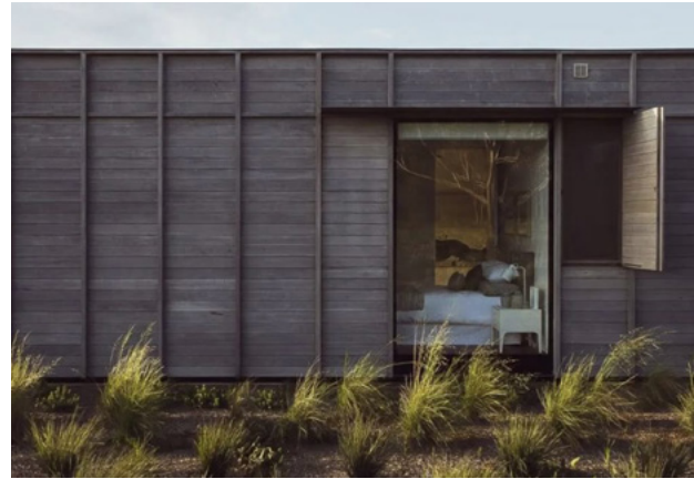
Timber weatherboards with raised batten detail
