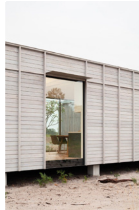
Timber weatherboards with raised batten detail
