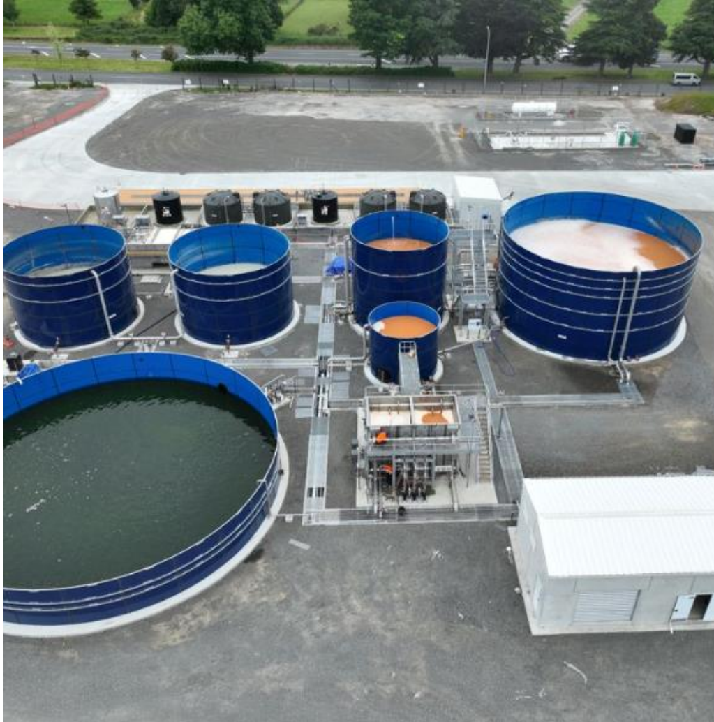
Figure 17 - Bolted Steel Panel Tanks on an Apex Designed and Built WwTP for a dairy site. The Milldale site will make use of a similar style of tanks as those coloured blue for the aeration and post-anoxic tank, the other equipment is unrelated to the Milldale sites.
