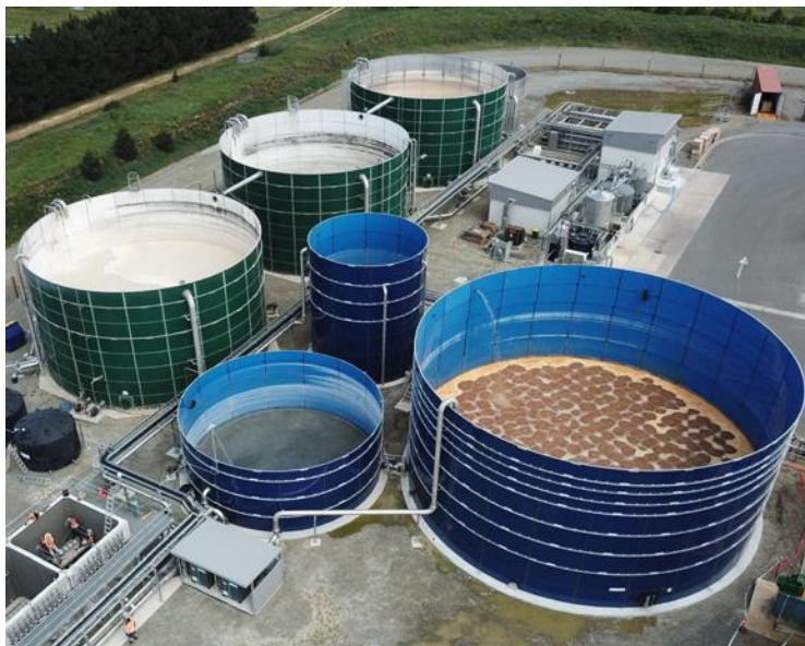
Figure 37 - An Aeration Tank in Action (Large Blue Tank on right) The aeration tank at Milldale will operate in a similar manner to this tank. All other vessels shown are unrelated to the Milldale site.
