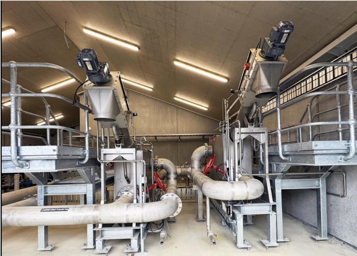
Figure 36 - Fine and Coarse Inlet Screens at a treatment plant designed and built by Apex Water
