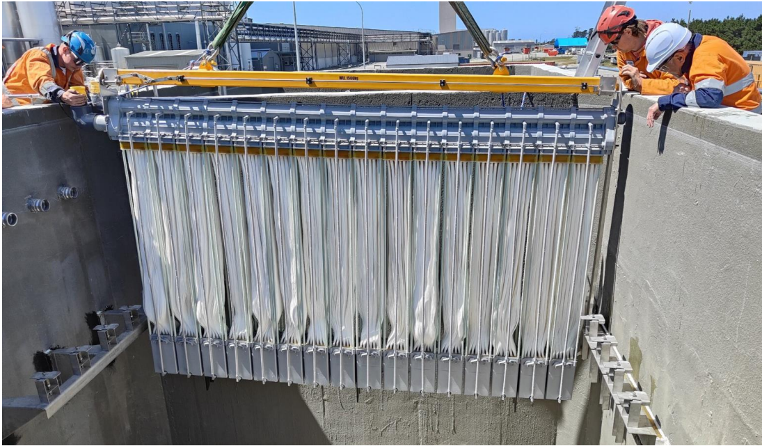
Figure 18 - A Hollow Fibre MBR Membrane Module on an Apex Wastewater treatment plant
