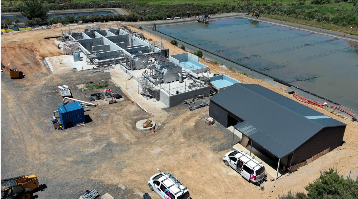
Figure 31 - Watercare Raglan MBR-MABR Designed and Built by Apex Water. This is being constructed on the site of an existing pond based WWTP. The Milldale site does not include any pond based treatment steps.
