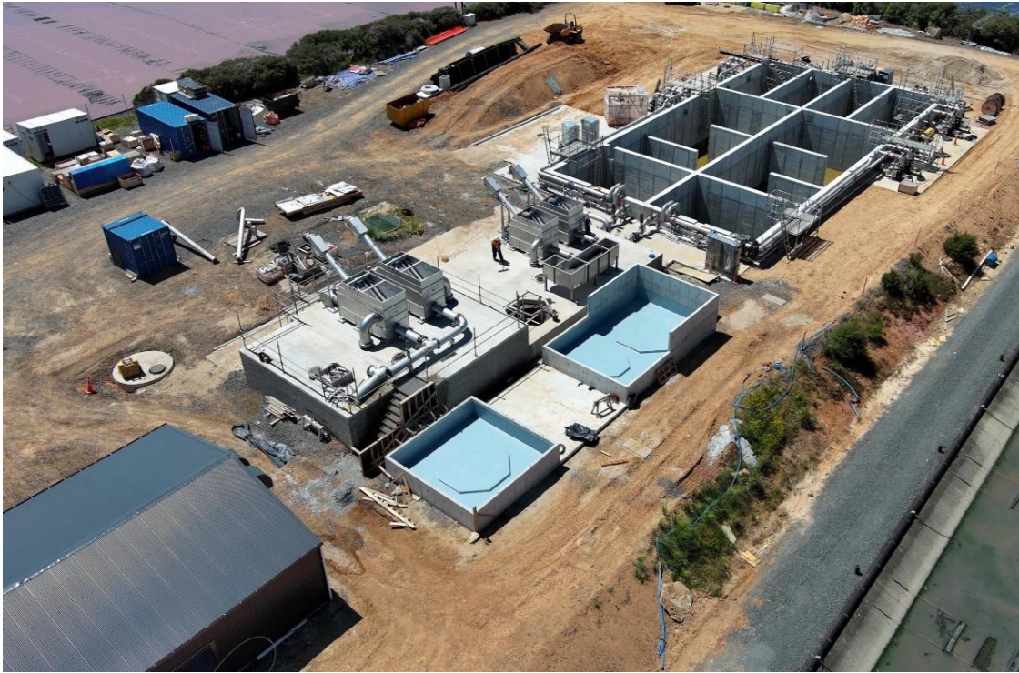
Figure 28 - Watercare Raglan MBR/MABR WwTP. Designed and under construction by Apex Water. This is a broadly similar process however it is not designed to be modular and hence the biological treatment tanks are made of concrete and buried. Milldale will have above ground modular, steel treatment tanks.
