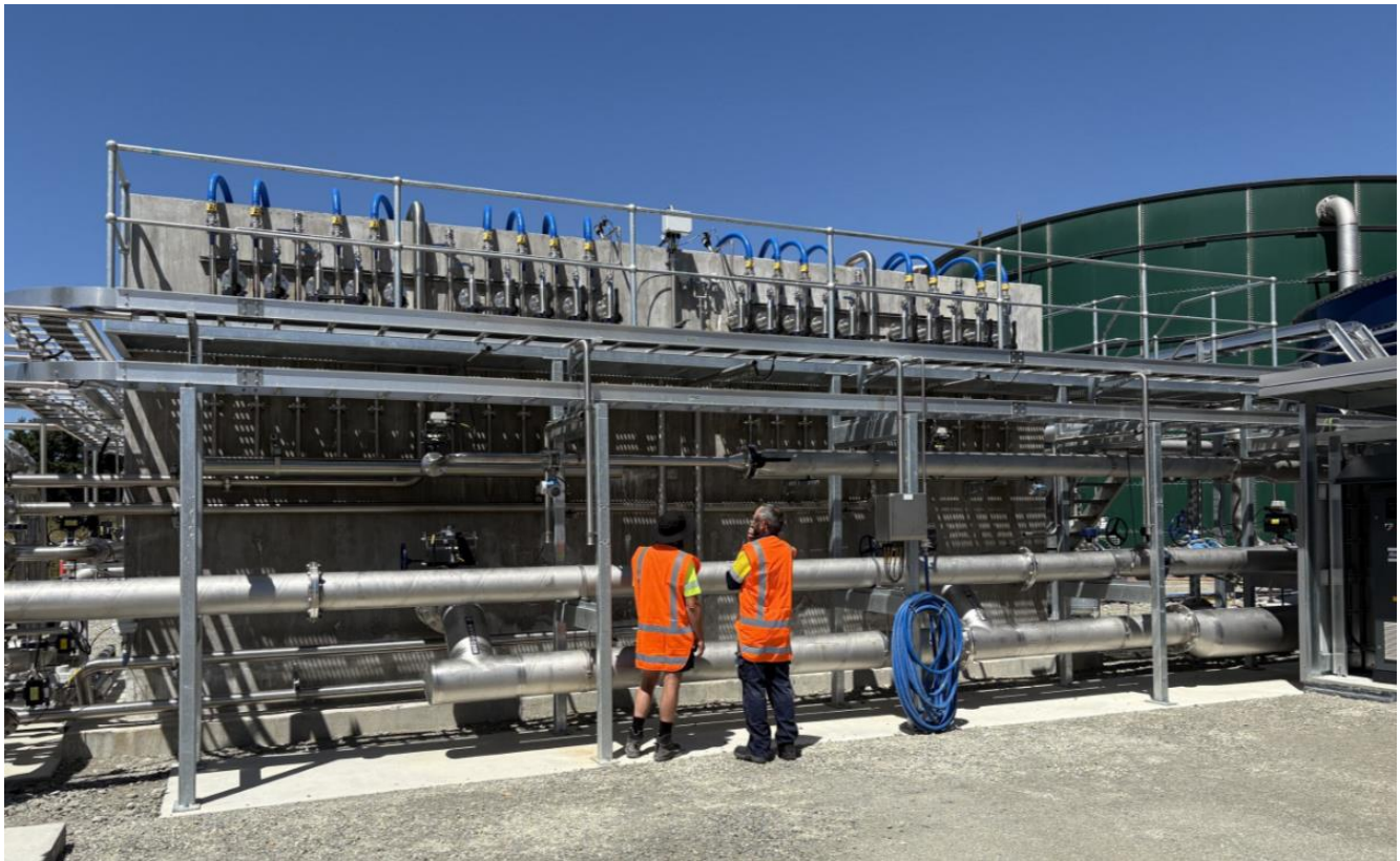
Figure 27 - The membrane tank of an MBR treatment plant designed and built but Apex Water. The Milldale site will make use of above ground tanks like those shown, but in steel.
