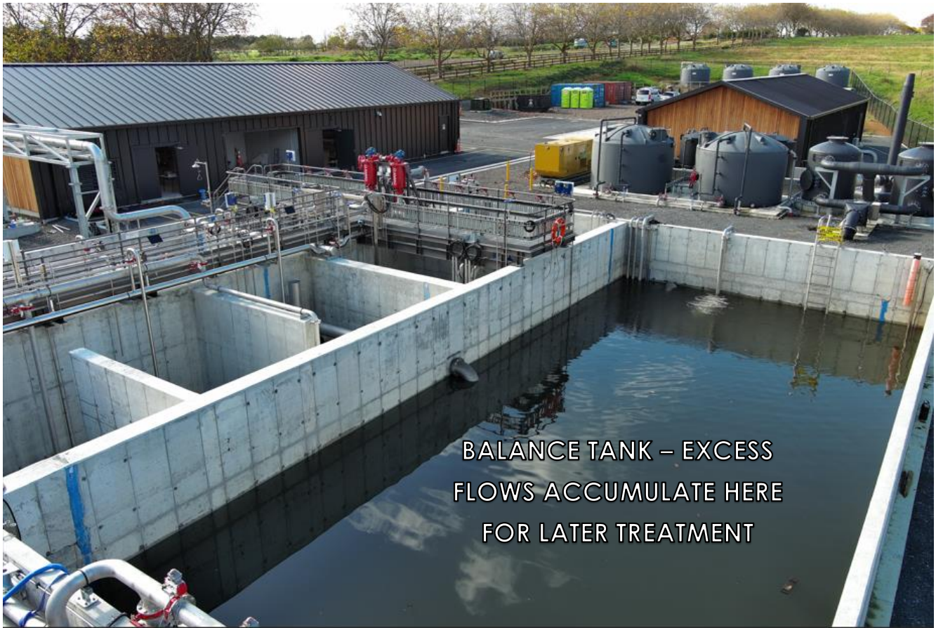
Figure 23 - A MBR WwTP with Flow Balancing. The Milldale site does not require any flow balancing
