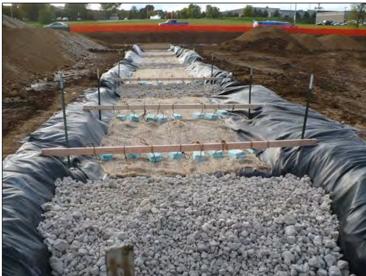
Figure 1 Tethered flock blocks with check dam system 1
