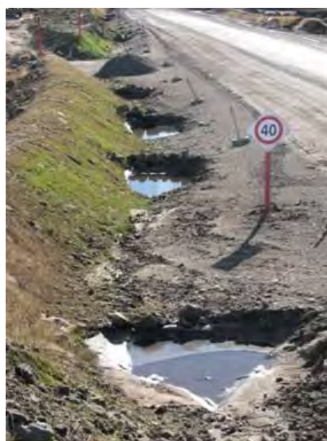
Figure 15. Roadside check dams at Stockton Mine.
