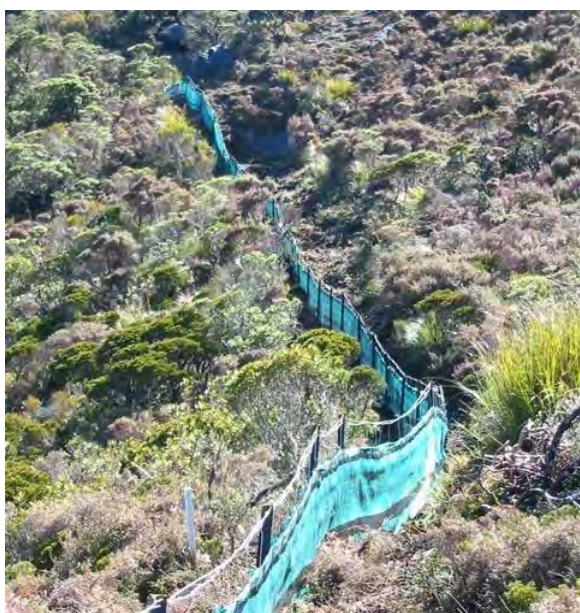
Figure 14. Silt fence installed prior to mining.
