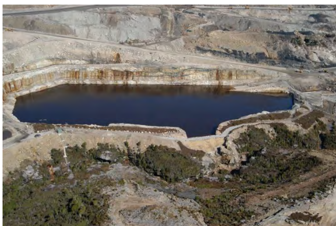
Figure 19. Aerial view of the Mangatini Sump.
