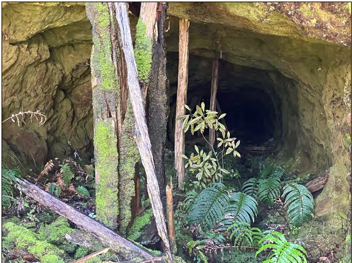
Photograph 8: BTM photograph taken 18 October 2023. Example of an adit in the historic underground workings. Adit roof propped with timber poles.
