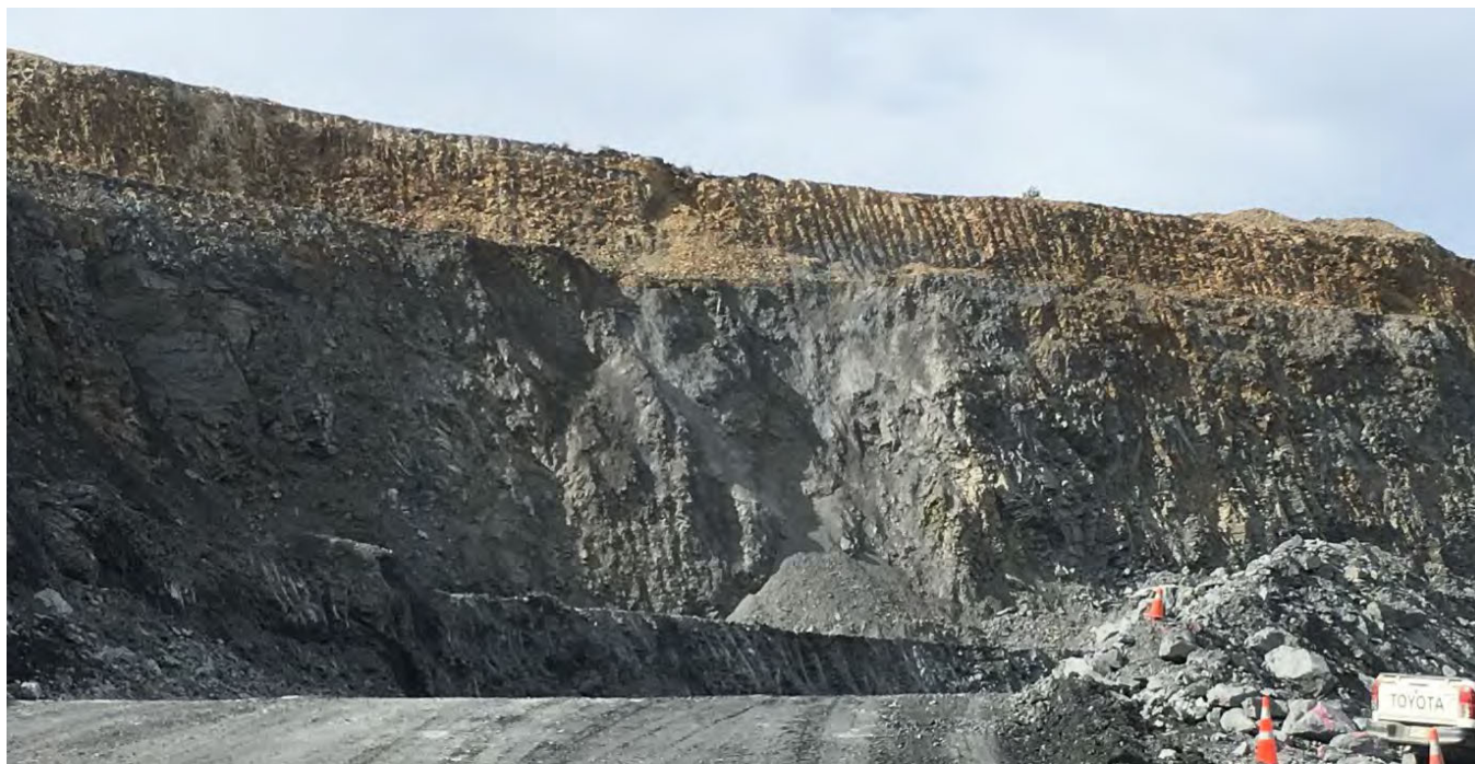
Inset 11: Coronation Pit Stage 2 – eastern wall of the ‘southern limb’. The 22.5 m high batters have not performed well in this rock mass.
