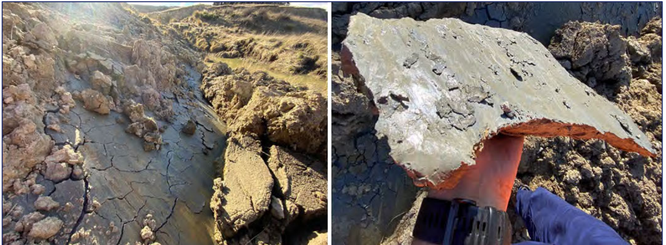
Inset 5: Example of the FF surface condition as exposed in the upper Frasers West headscarp. The sliding surface is described as slickensided and undulous, comprising high plasticity moist firm clay.
