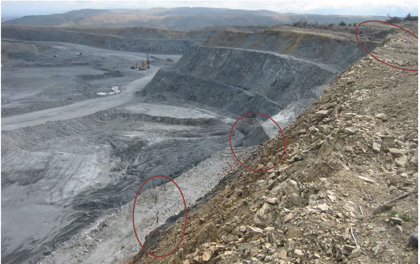
Inset 9: South-eastern wall of Coronation Pit Stage 1, 2015. Wedge failures and cracking formed along north-south trending, westerly dipping faults.
