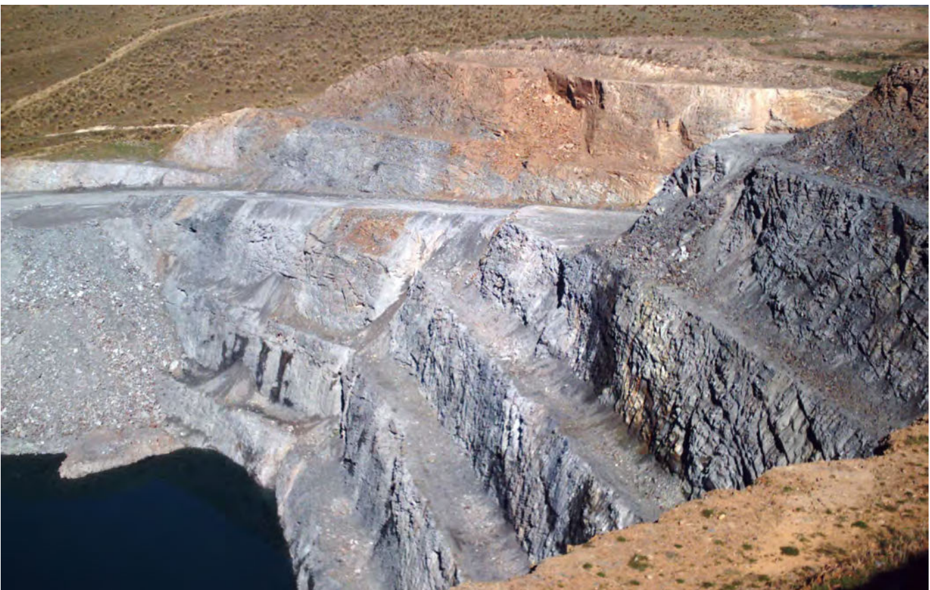
Inset 26: January 2009 – north wall. Photo taken from crest looking west. Pre-split 75° batters. Note joint bound wedges.
