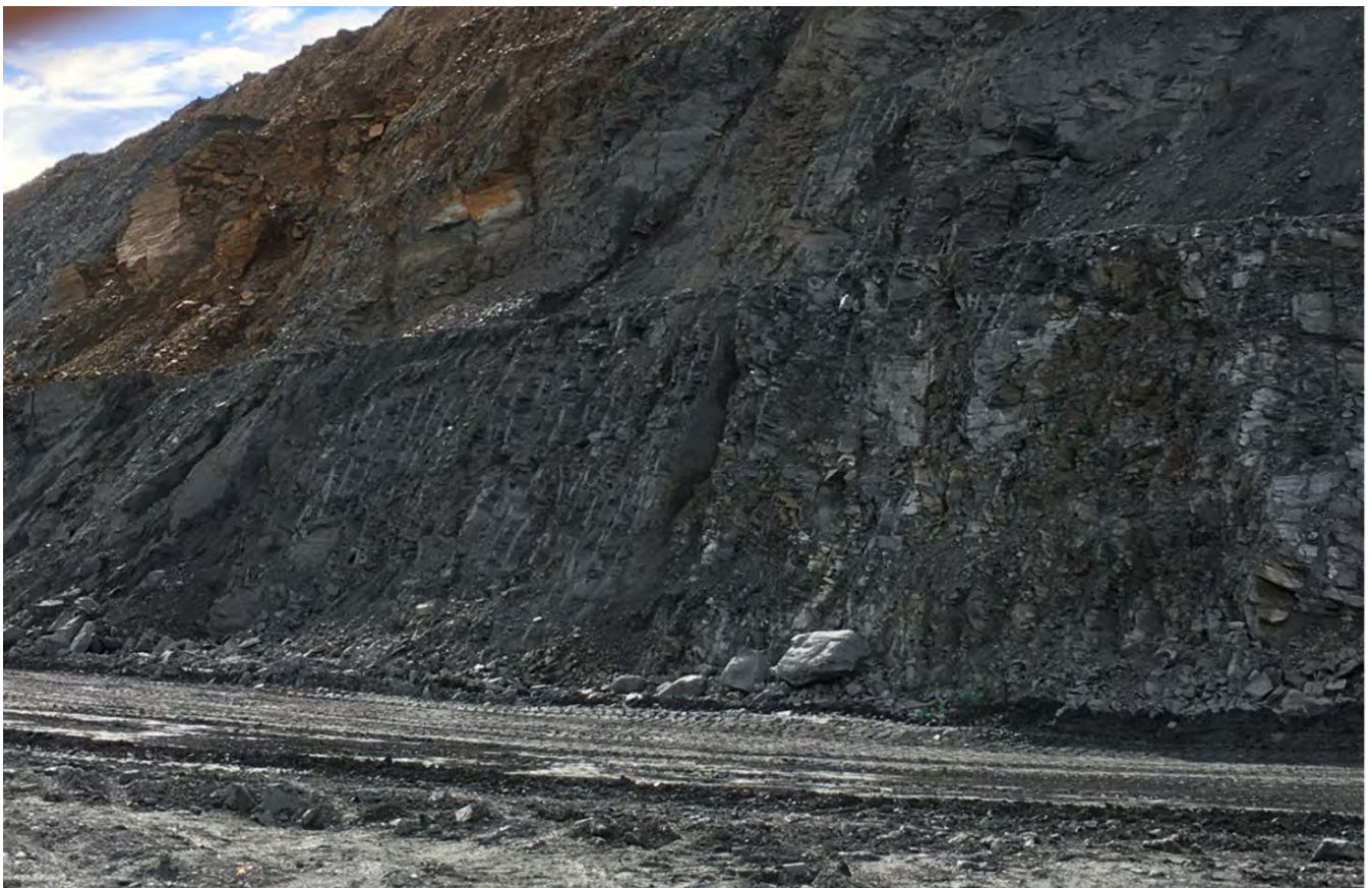
Inset 10: Coronation Pit Stage 2 – eastern wall immediately south of the ‘fish bowl’. Westerly dipping faults can be seen outcropping at 270°.
