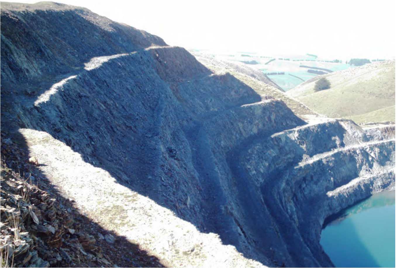
Inset 25: January 2009 - east wall taken from crest facing south. Berms are relatively clean.
