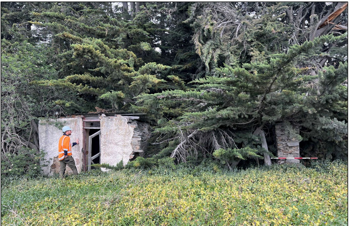
Figure 28. Stone outbuilding, looking south-west.
