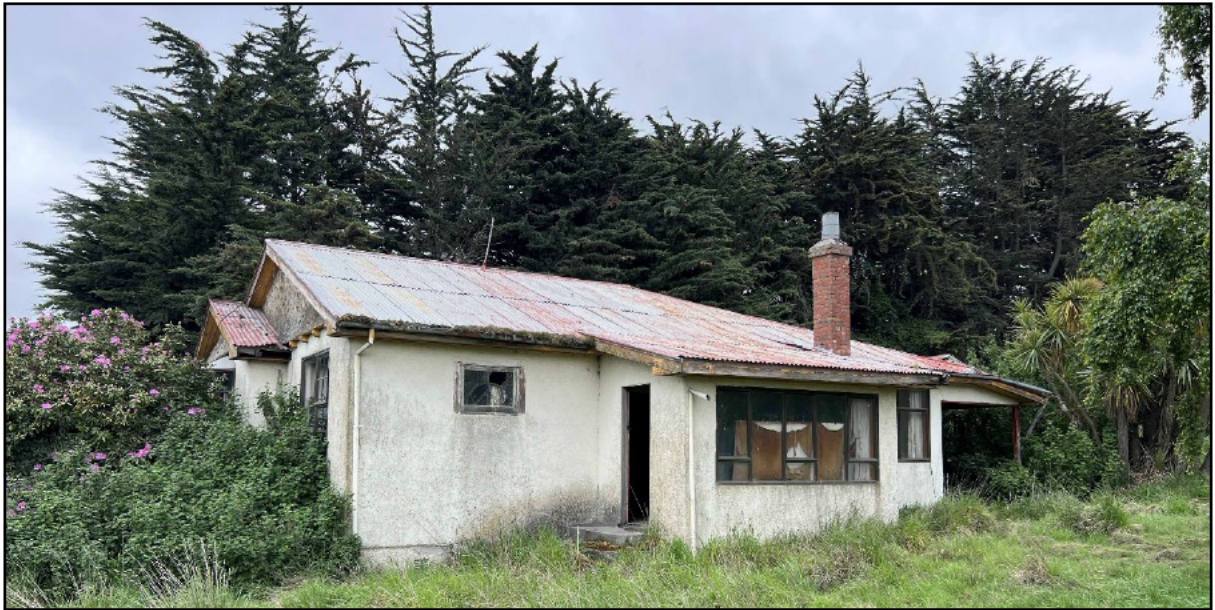
Figure 25. Innes house, looking west.
