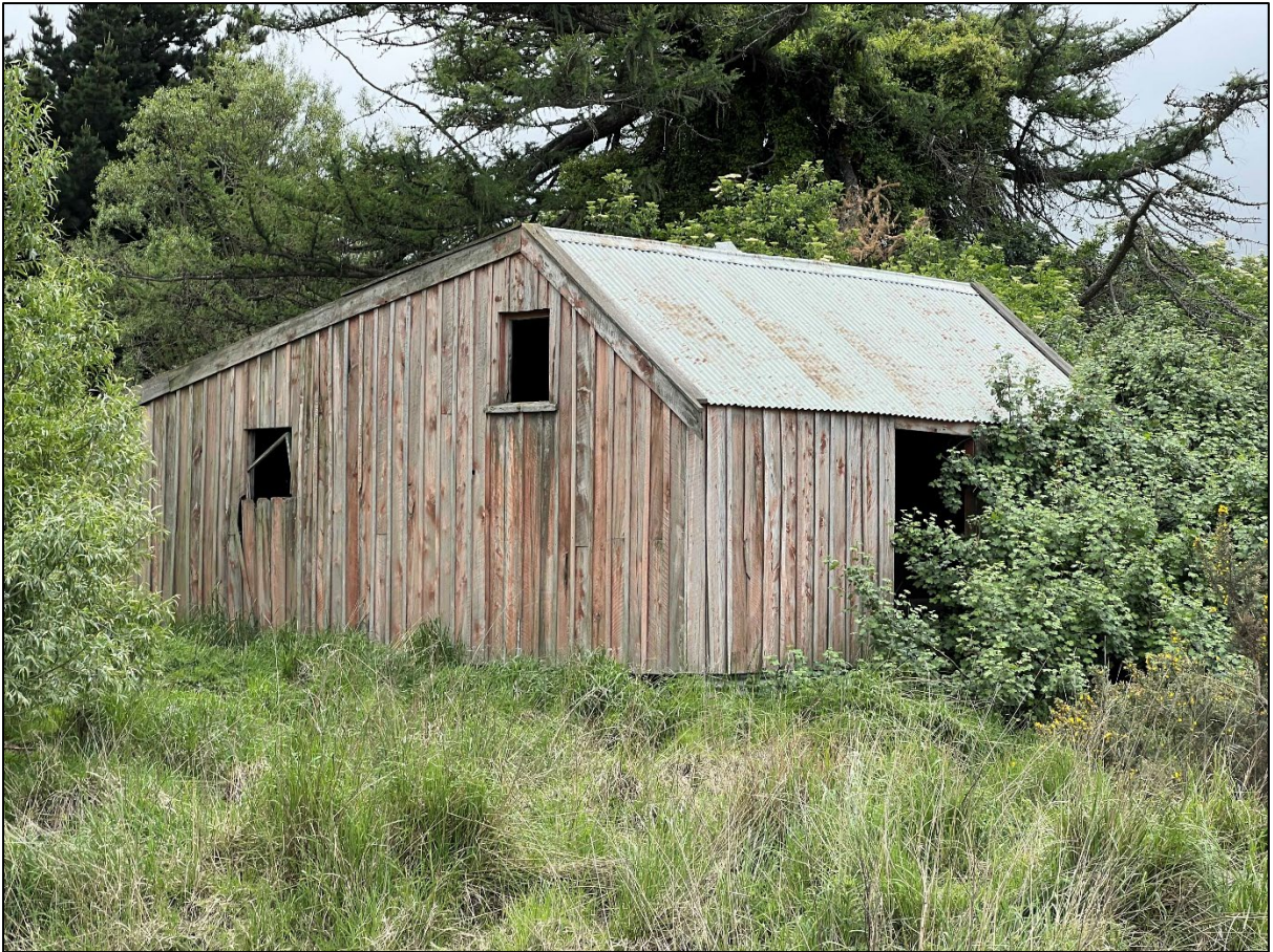
Figure 27. Shearing shed/barn, looking north.
