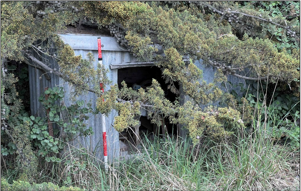
Figure 31. Pump house, looking west.
