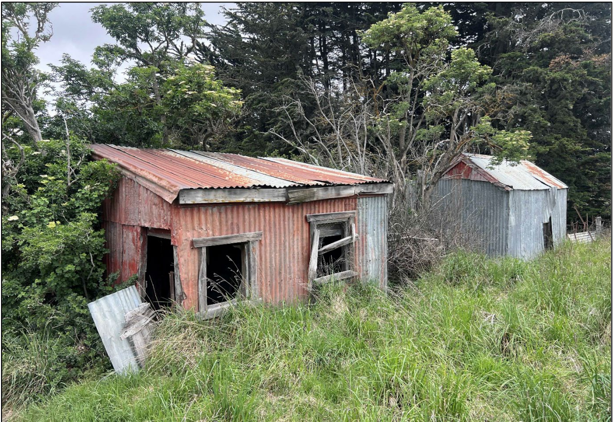
Figure 30. Outbuilding F, looking south.
