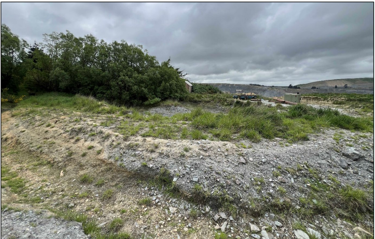
Figure 36. Modern dam, looking north.
