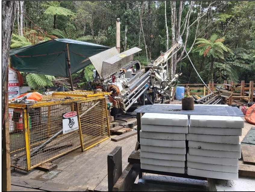
Figure 2-9: Typical Drilling Set Up (vertical drilling will be employed for shaft geotechnical investigation)
