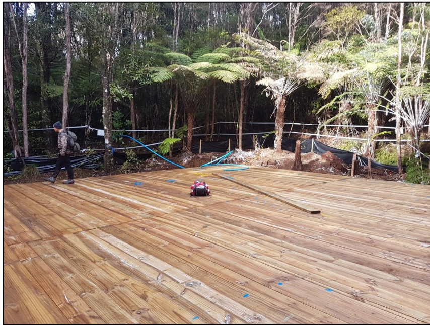
Figure 2-8: Typical Drilling Platform Construction
