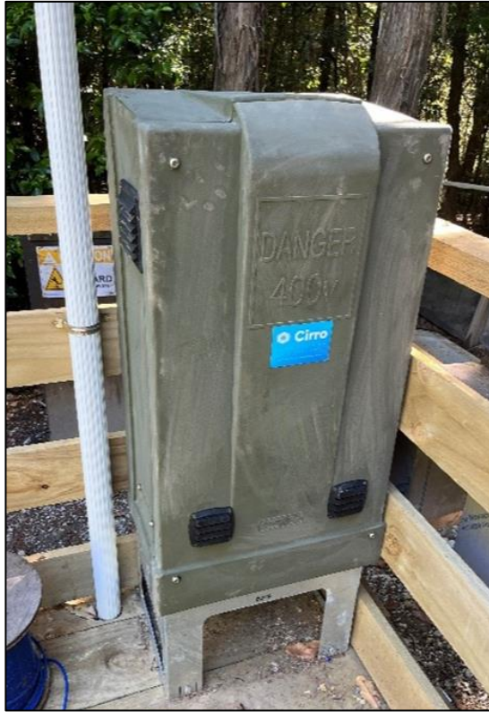
Figure 2-14: Example of Data Logger Box Installation after Piezometer Construction
