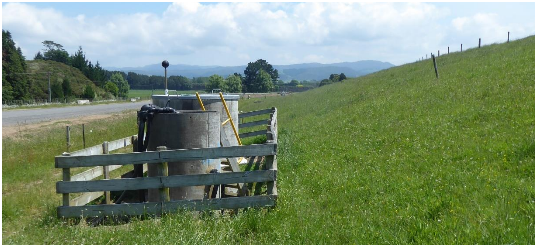
FIGURE 23: COLLECTION SUMP T18 AT TOE OF STORAGE 1A
