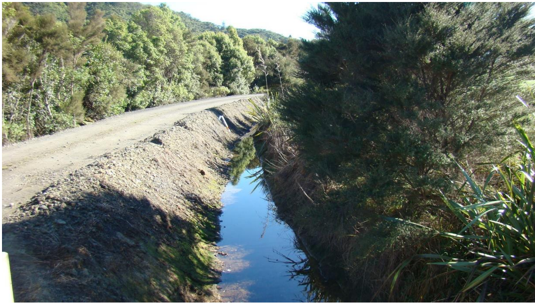
FIGURE 20: PERIMETER DRAIN BESIDE PERIMETER ROAD SOUTHEAST SIDE OF STORAGE 2.
