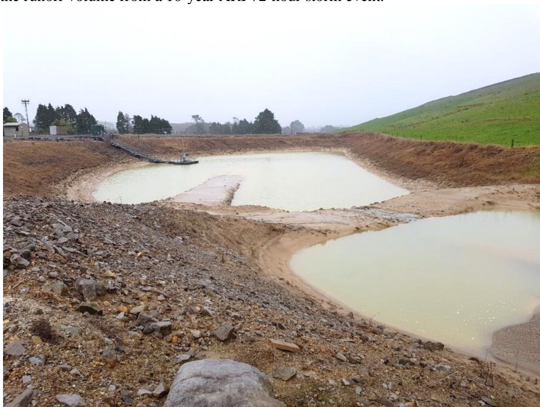
FIGURE 24: STORAGE 1A COLLECTION POND S5, WITH FOREBAY AND MAIN POND
