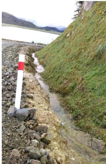
FIGURE 19: CLEAN WATER UPHILL DIVERSION DRAIN - NORTH
