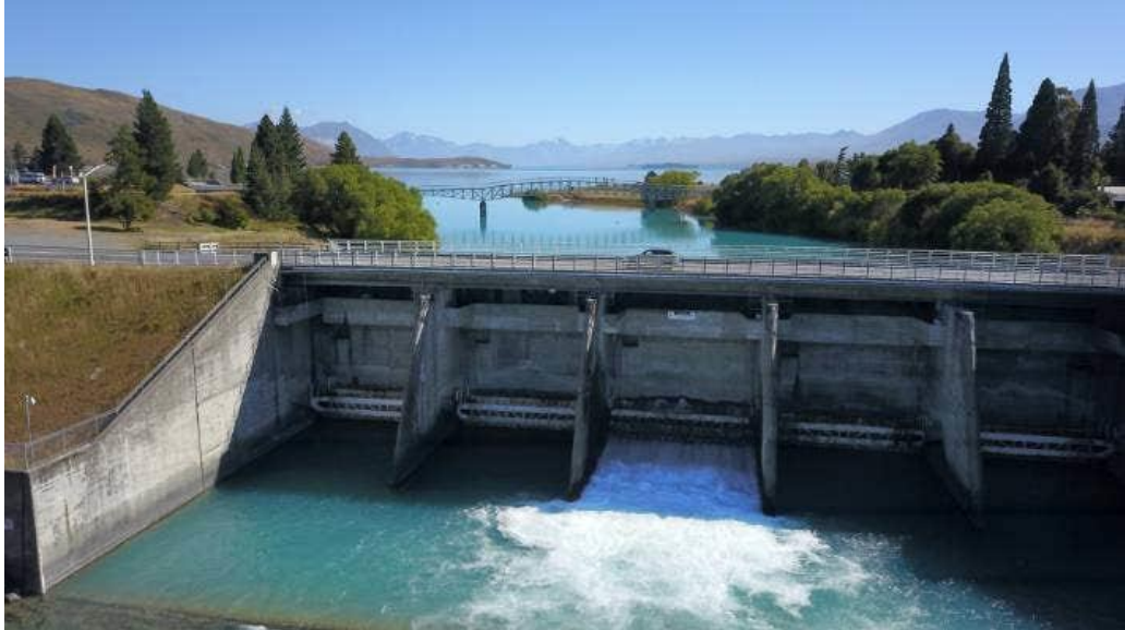
Figure 14: Gate 16 Radial Gates
