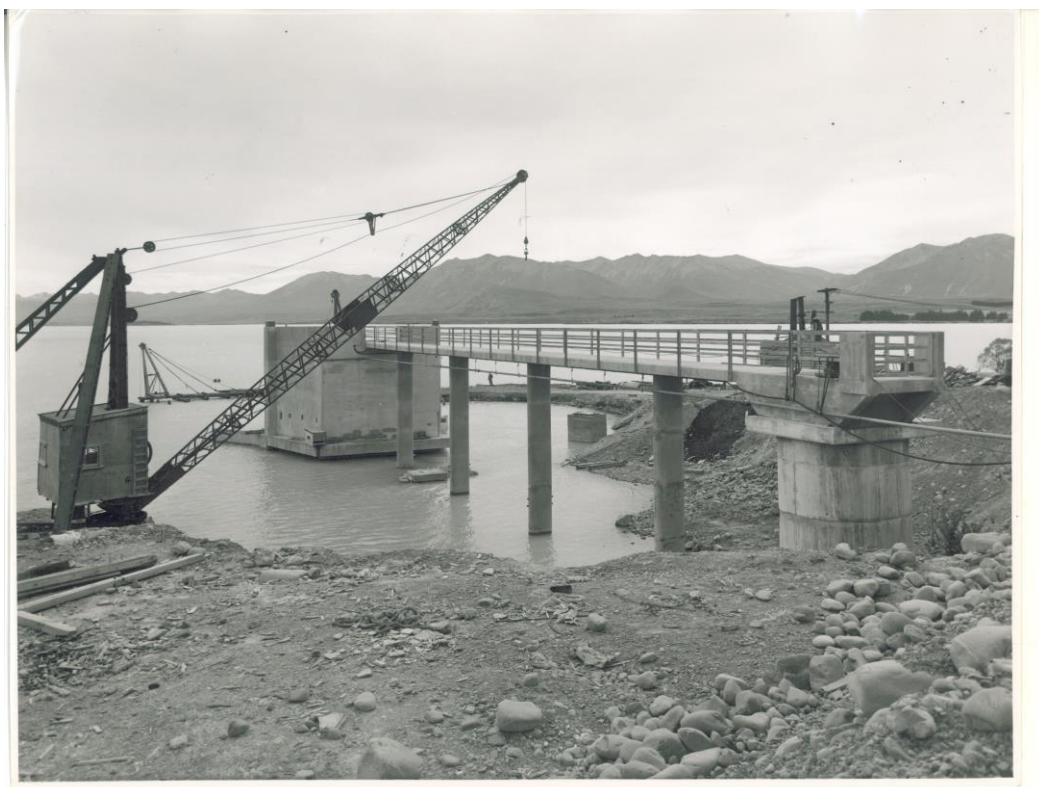
Figure 6: Tekapo Intake Nearing Completion (1952)
