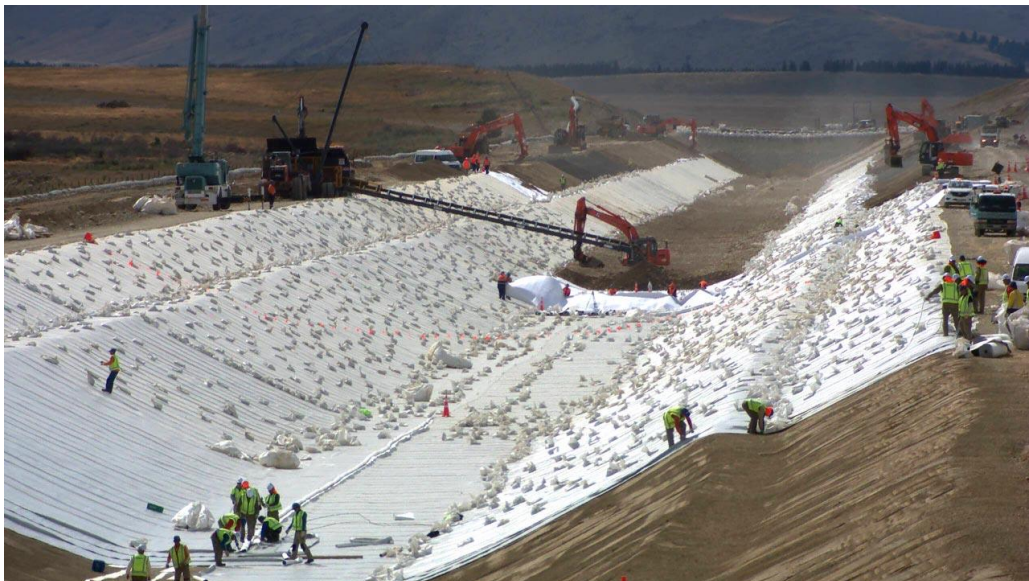
Figure 24: Tekapo Canal Lining Works
