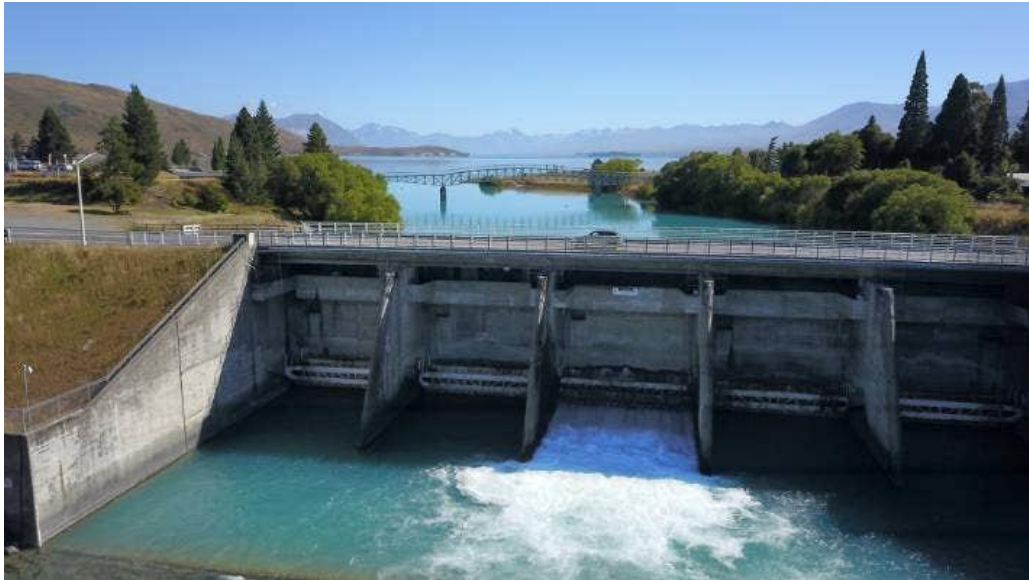
Figure 14: Gate 16 Radial Gates
