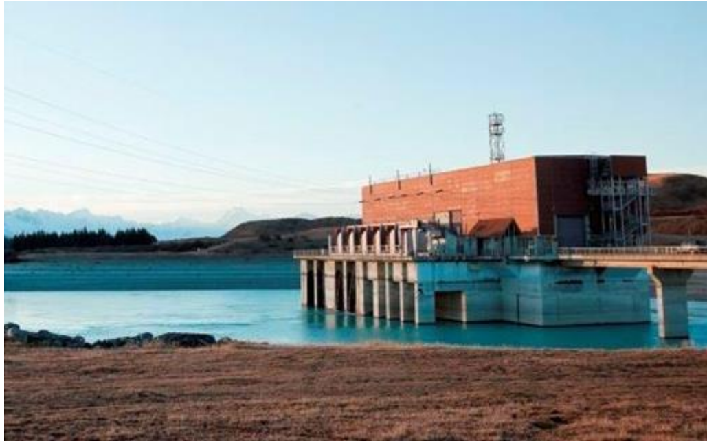
Figure 25: Tekapo B Power Station
