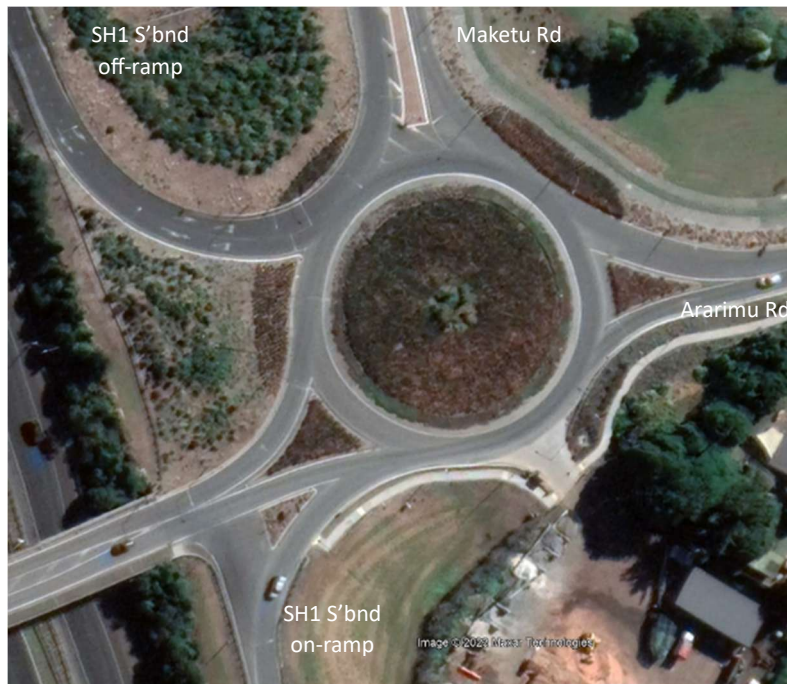
Figure 8: Intersection of Maketu Road and Ararimu Road (Image Source: Google Earth)
