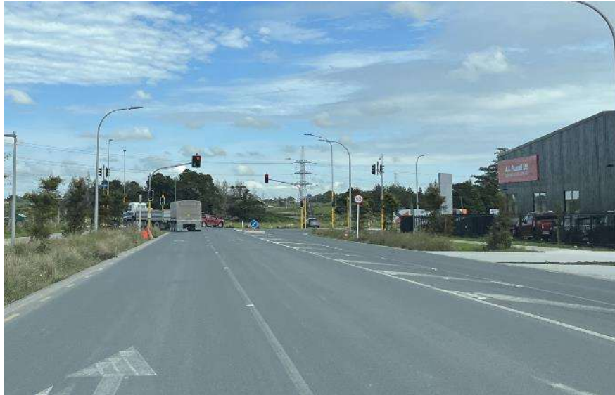
Figure 6: Intersection of Bill Stevenson Drive and Maketu Road (eastern approach)
