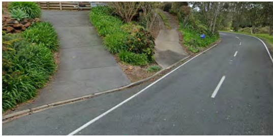
Driveways near Ramp on Rangitane Loop Road
