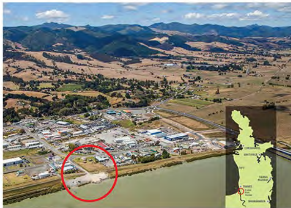
Kopu Boat Ramp, Off Quay Street, Kopu
