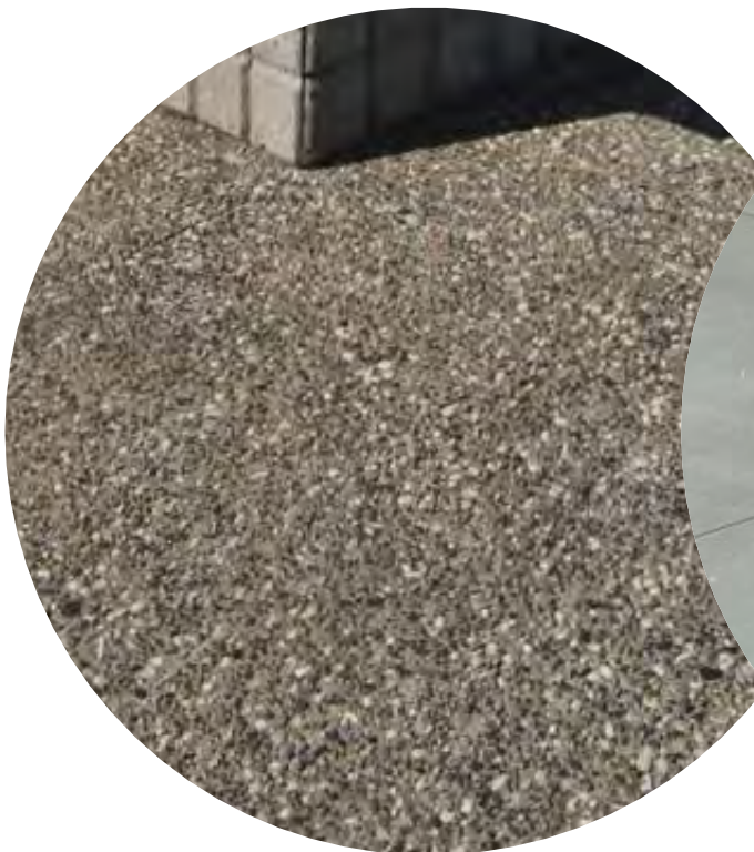
Exposed aggregate concrete
