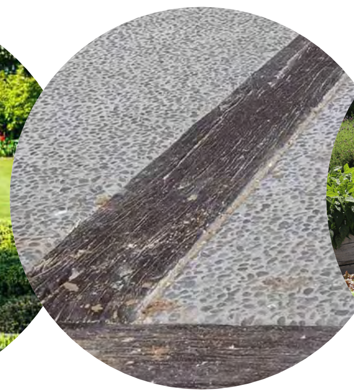
Timber Sleeper in Concrete
