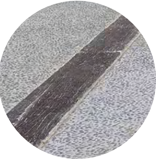
Sleeper in Concrete
