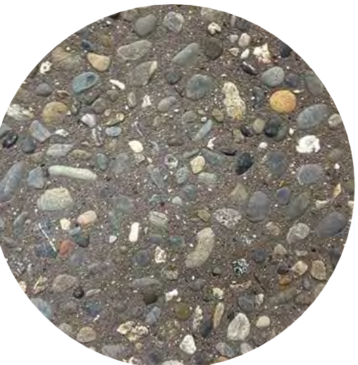
Exposed Aggregate Concrete
