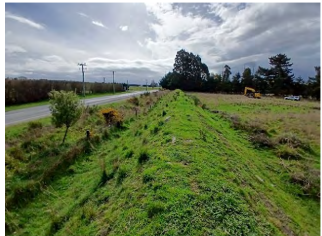
Soil bund along S boundary, comprising construction debris/non-engineered fill
