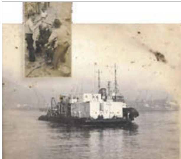
Figure 2—Barge 77—MDC's first production system
