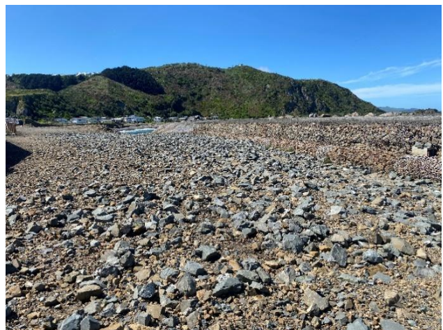
Photo 9. Inside of the seawall (looking east) at Moa Point showing a barren
