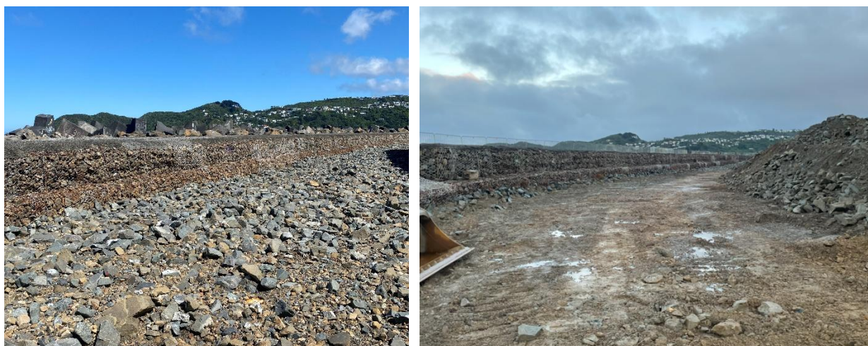
Photo 4. (L) Inner seawall and wave trap area seawall looking east, photo taken October 2024; (R) photo taken July 2025 after maintenance works were undertaken.
