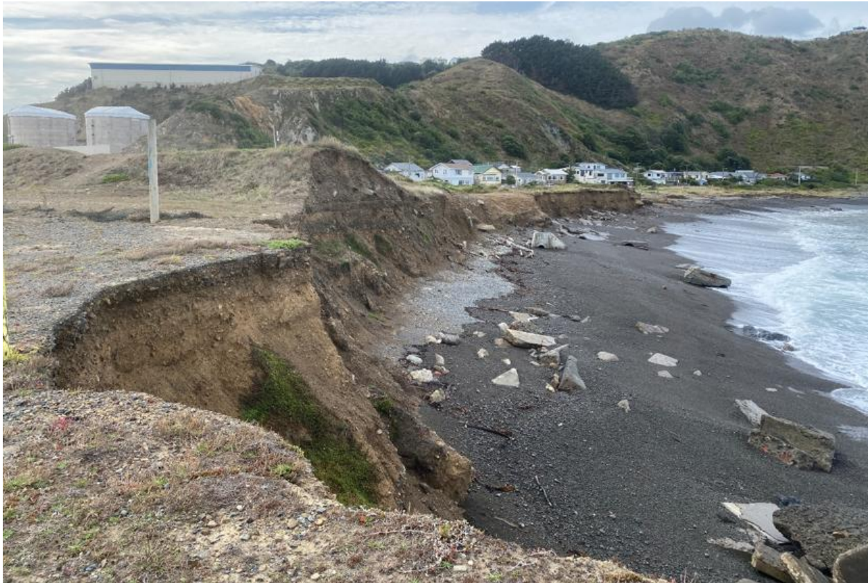
Photo 6. Looking east toward Moa Point beach, and the proposed eastern bank remediation site (2 April 2025). Note that current bank has eroded further since this image.
