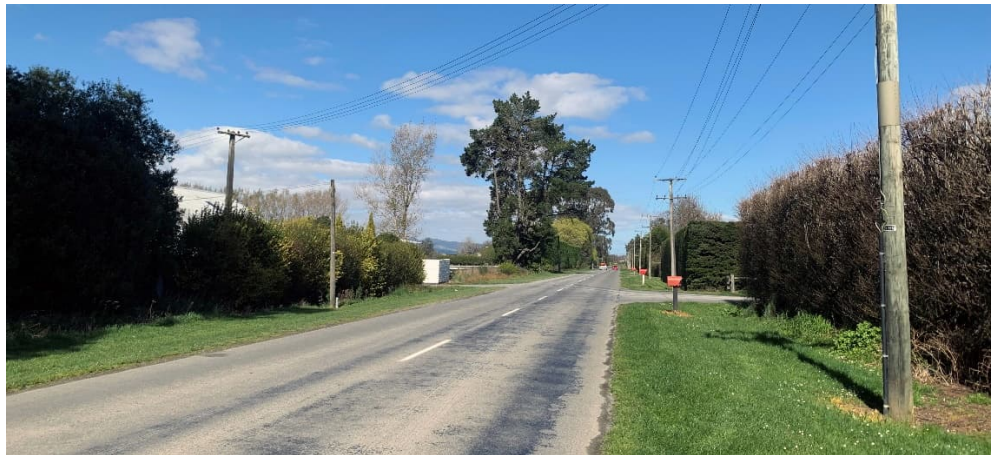
Figure 1 - Typical view looking south down Barters Road.
