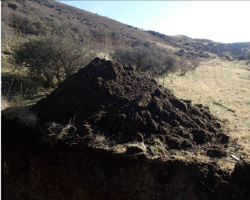
Spoil pile at end of excavation
