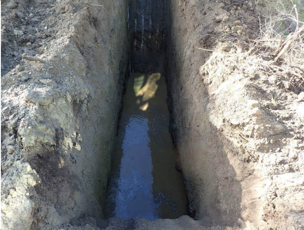
Testpit at completion. Max depth 5m
