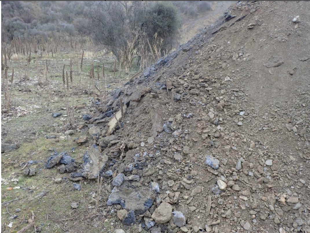
Spoil pile at end of excavation
