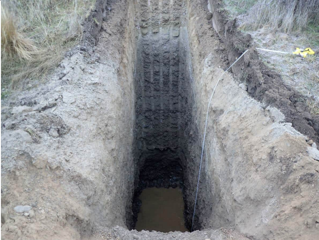
Testpit at completion. Max depth 7m
