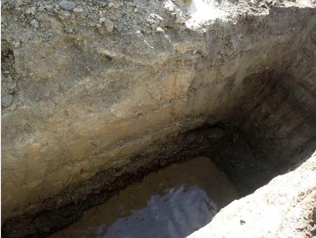
Testpit at completion. Max depth 6.5m
