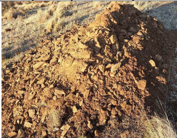
Spoil pile at end of excavation
