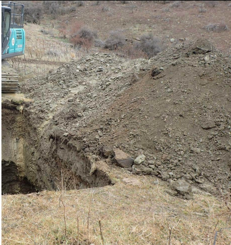
Spoil pile at end of excavation
