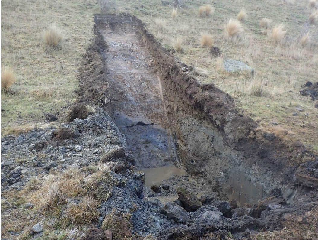
Testpit at completion. Max depth 7m
