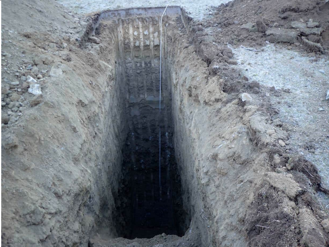
Testpit at completion. Max depth 7m
