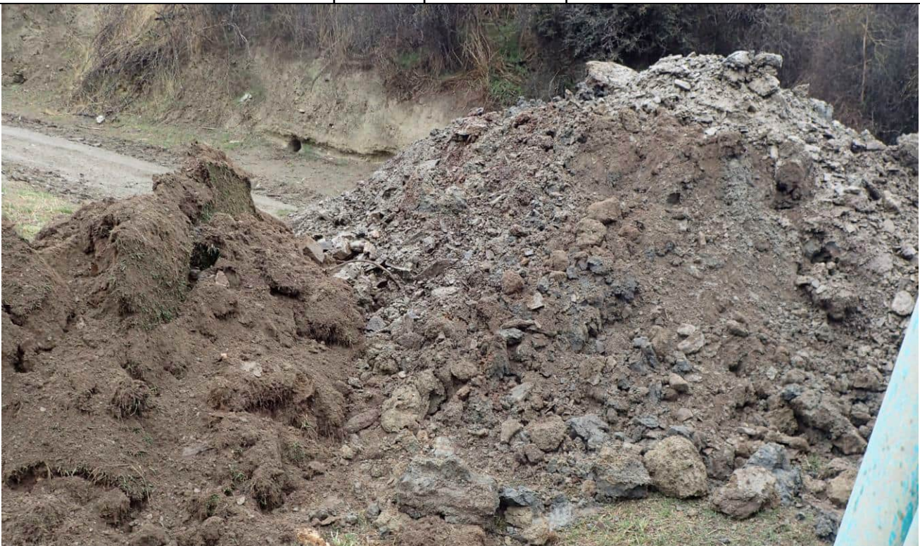
Spoil pile at end of excavation
