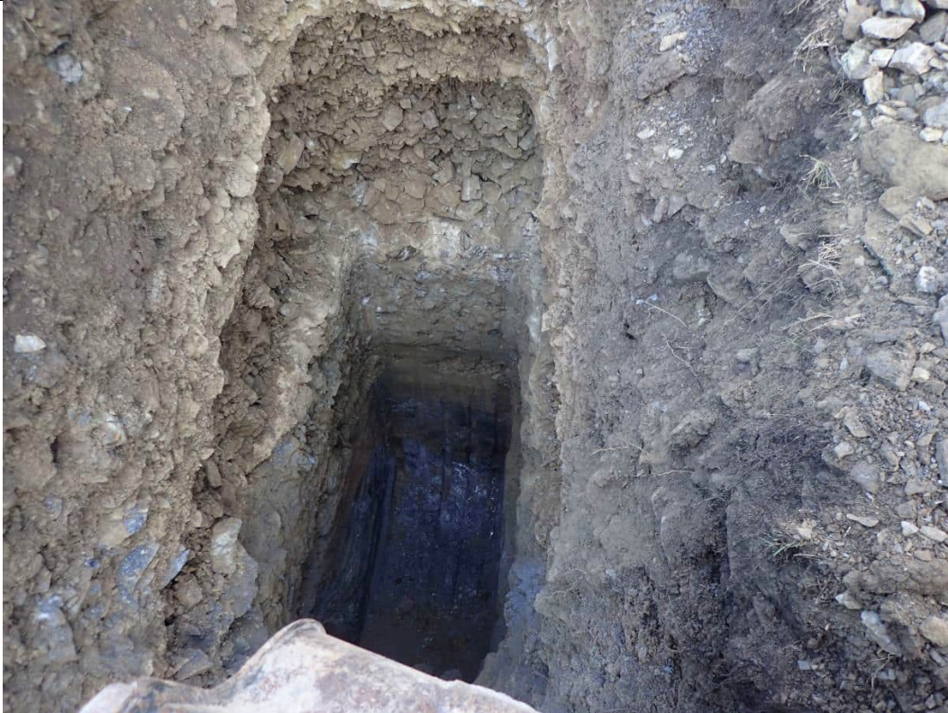
Testpit at completion. Max depth 6.5m
