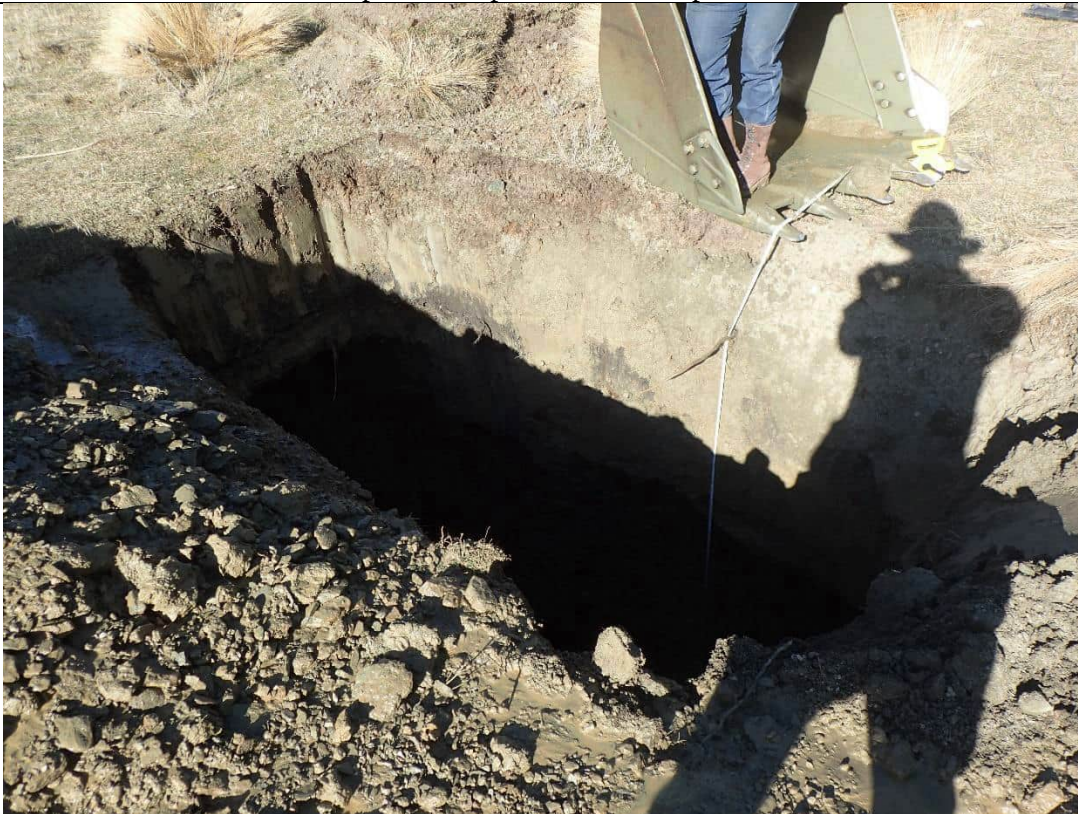
Spoil pile at end of excavation
