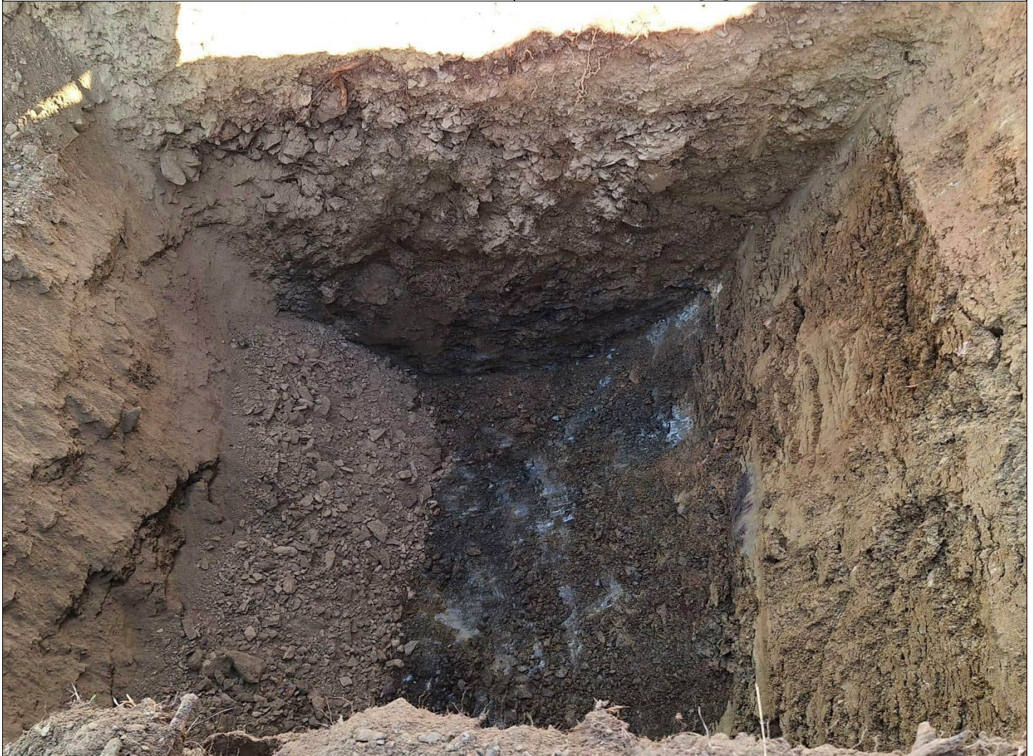
Testpit at completion. Max depth 2.4m
