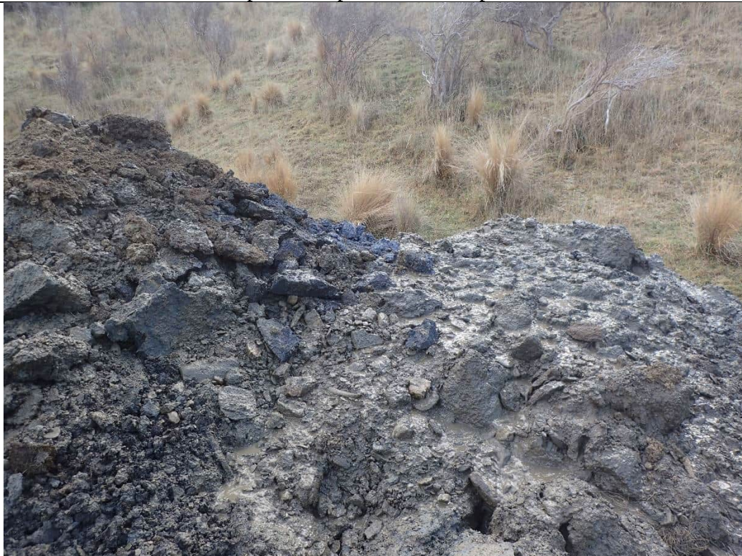
Spoil pile at end of excavation
