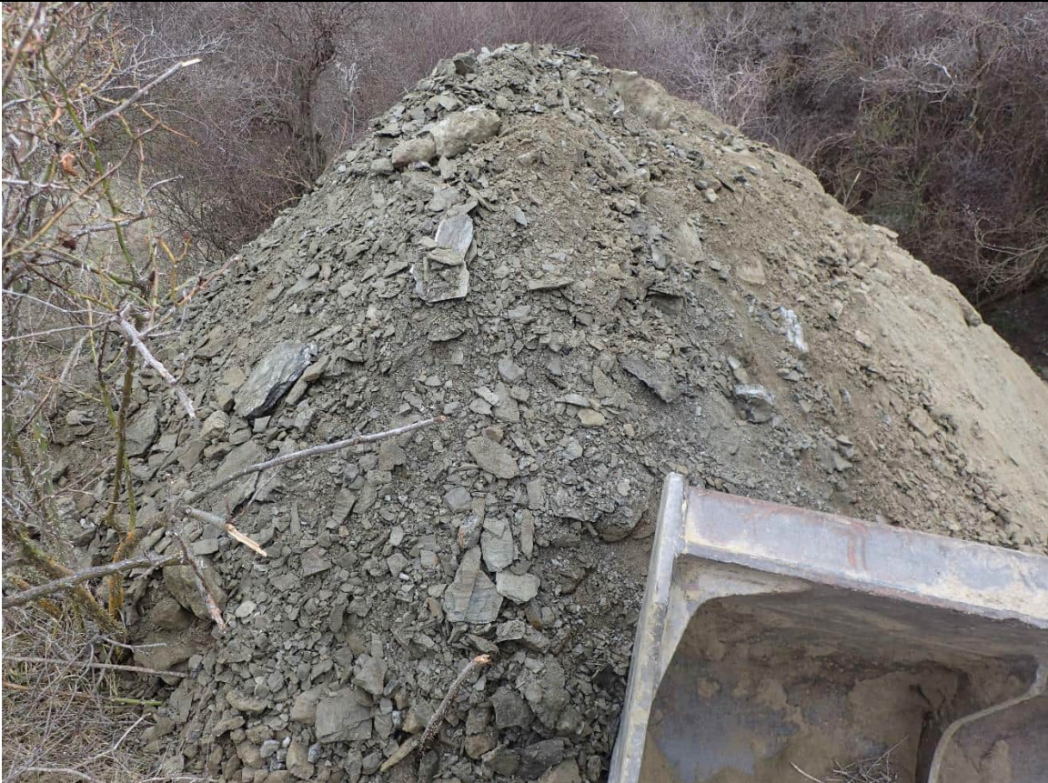
Spoil pile at end of excavation
