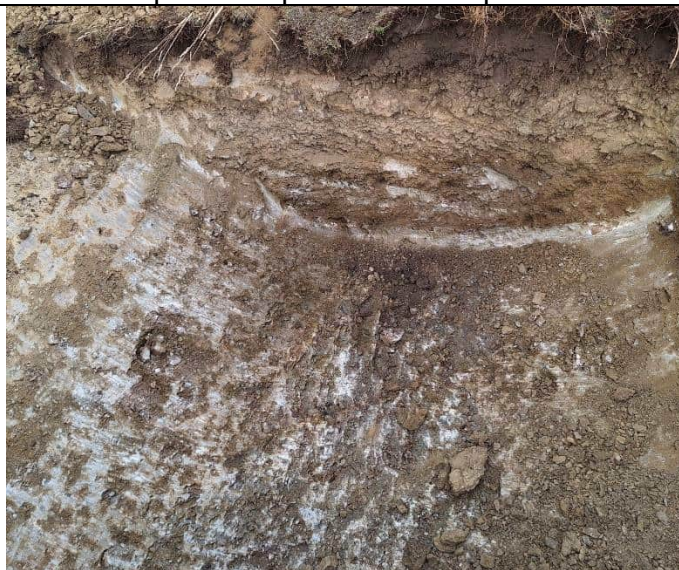
Spoil pile at end of excavation
