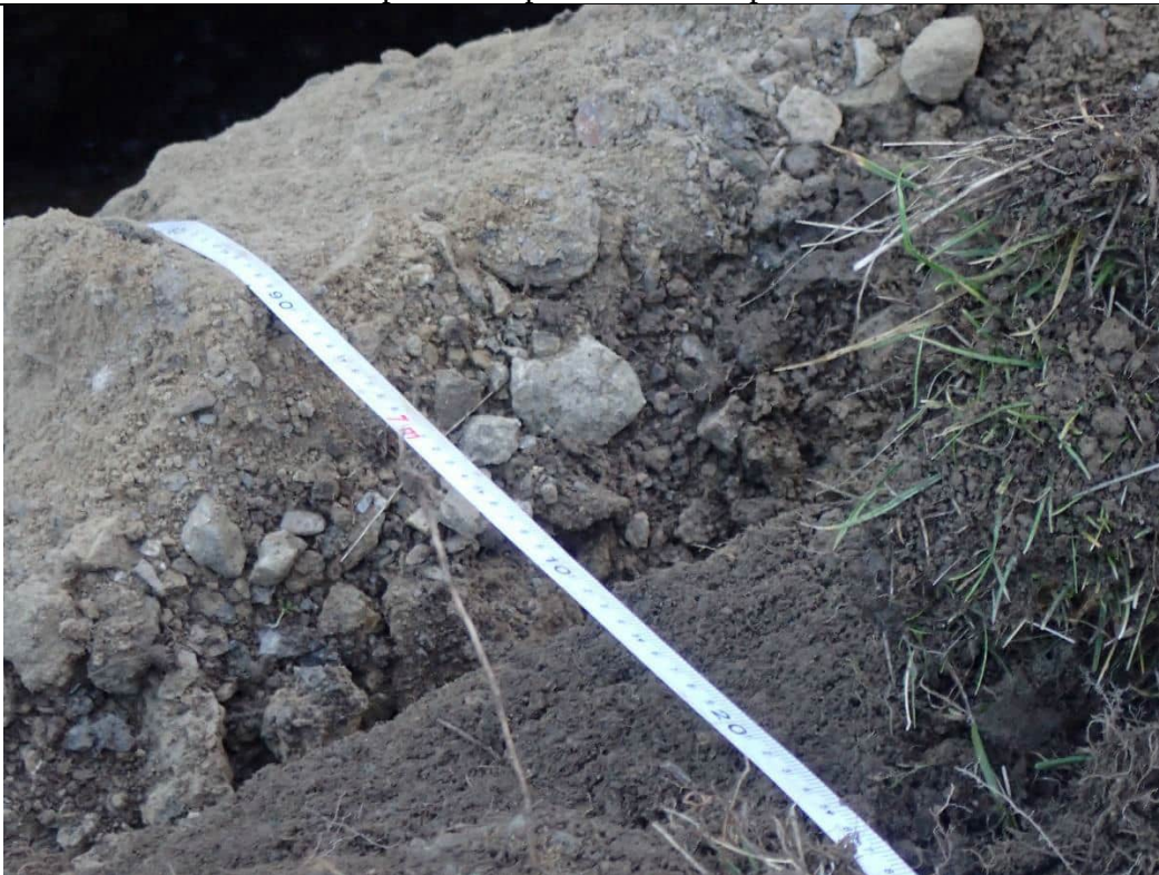
Spoil pile at end of excavation
