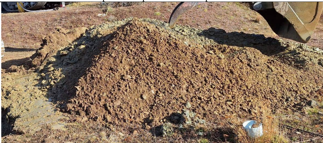
Spoil pile at end of excavation
