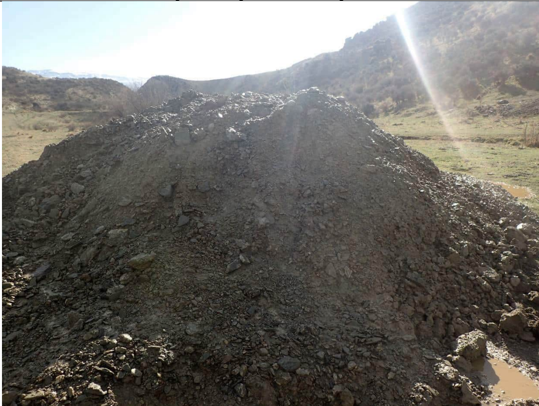
Spoil pile at end of excavation
