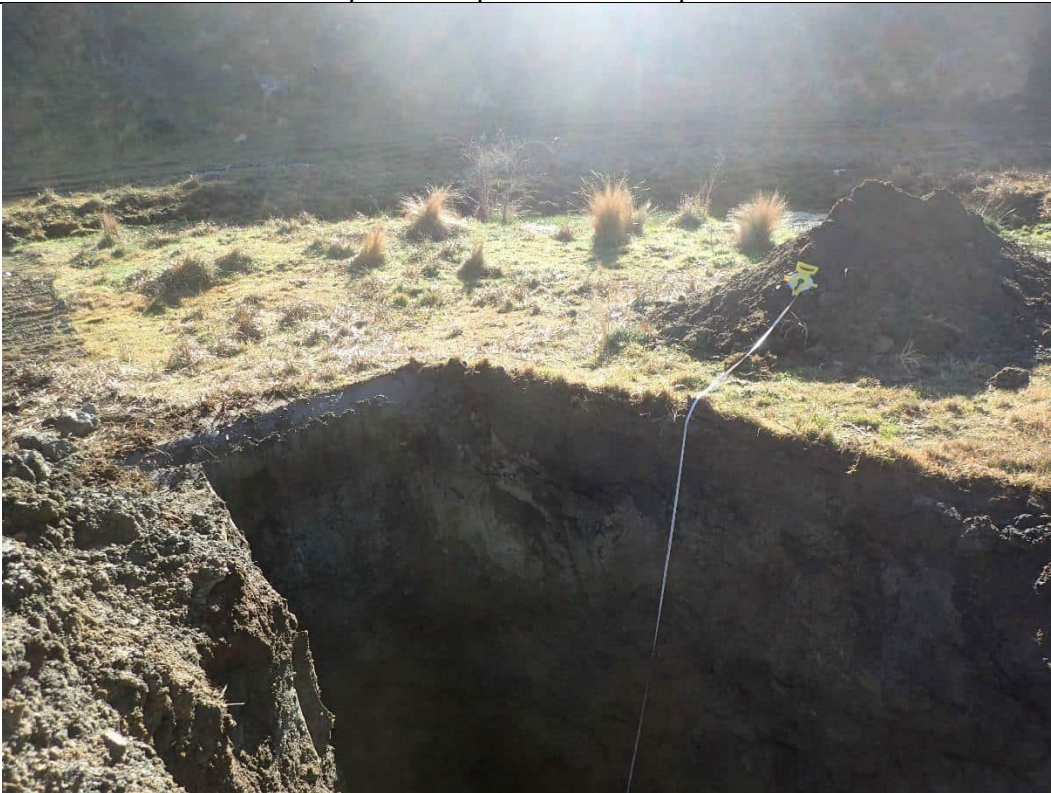
Spoil pile at end of excavation
