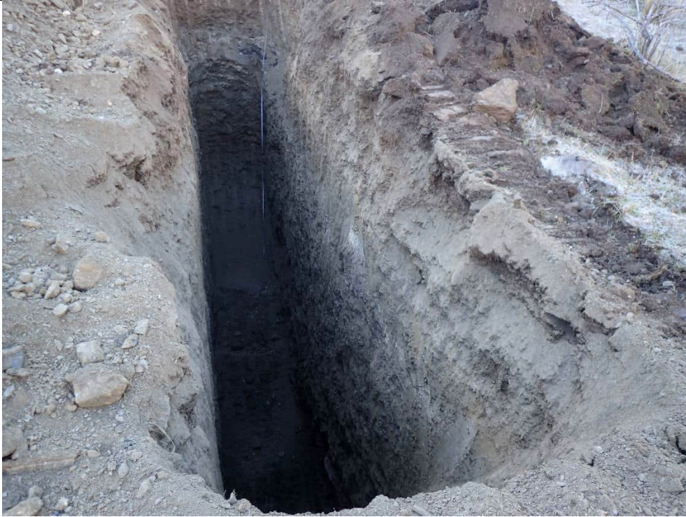
Testpit at completion. Max depth 6m
