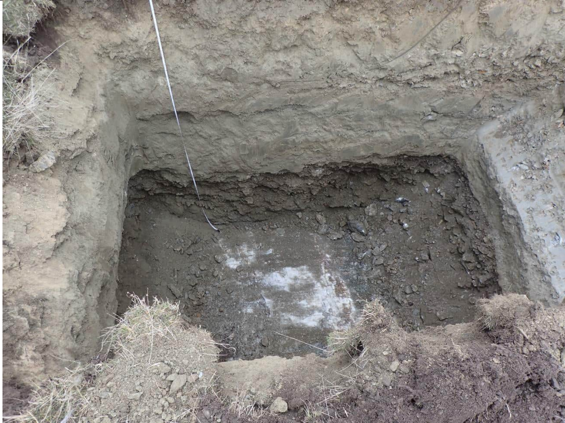
Testpit at completion. Max depth 4.1m
