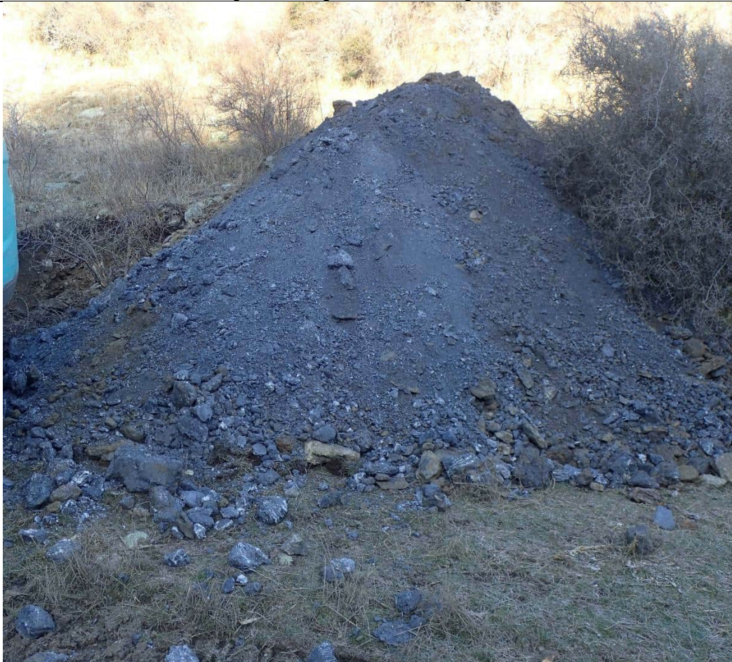
Spoil pile at end of excavation
