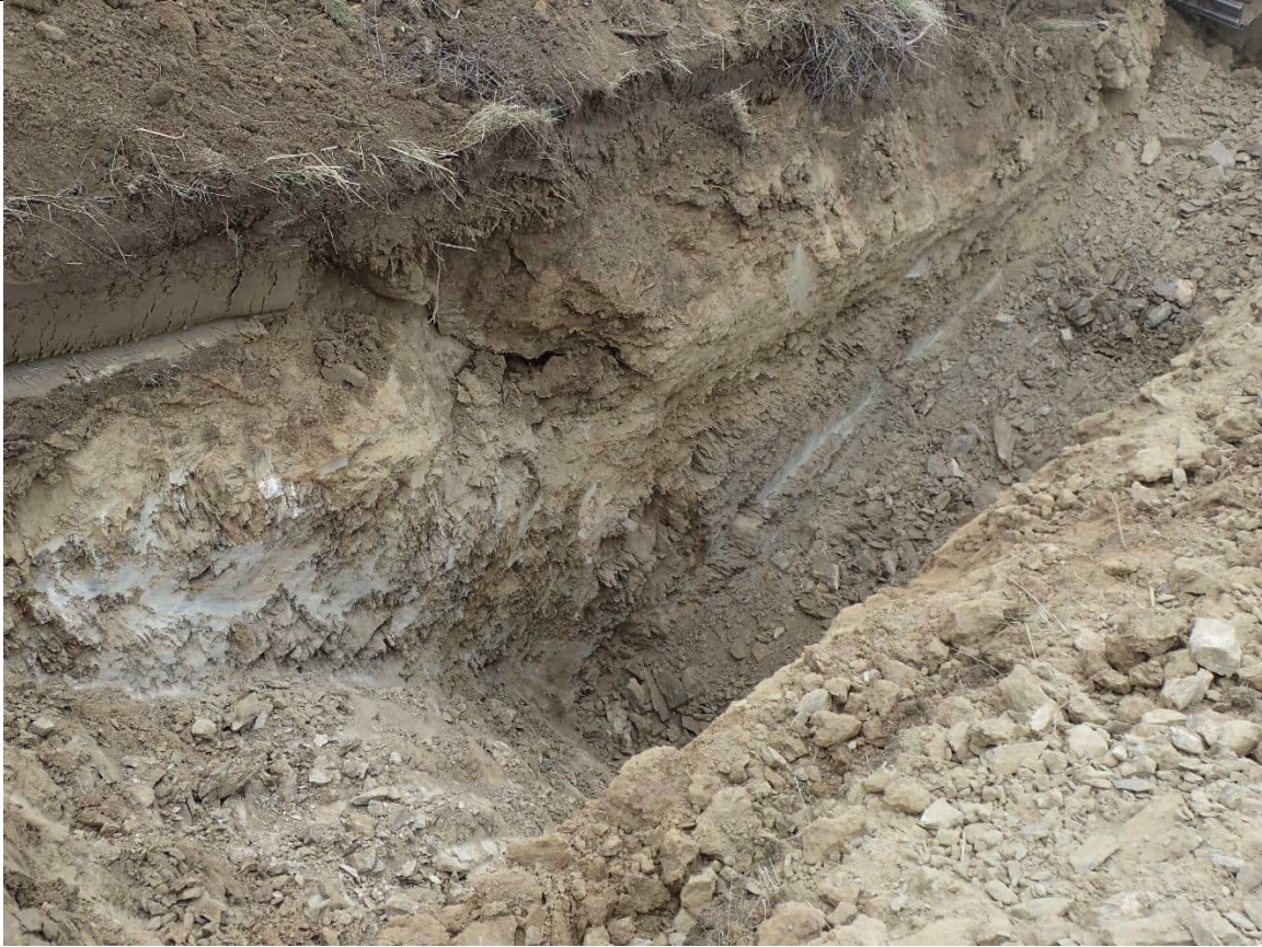
Testpit at completion. Max depth 3.5m
