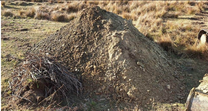
Spoil pile at end of excavation
