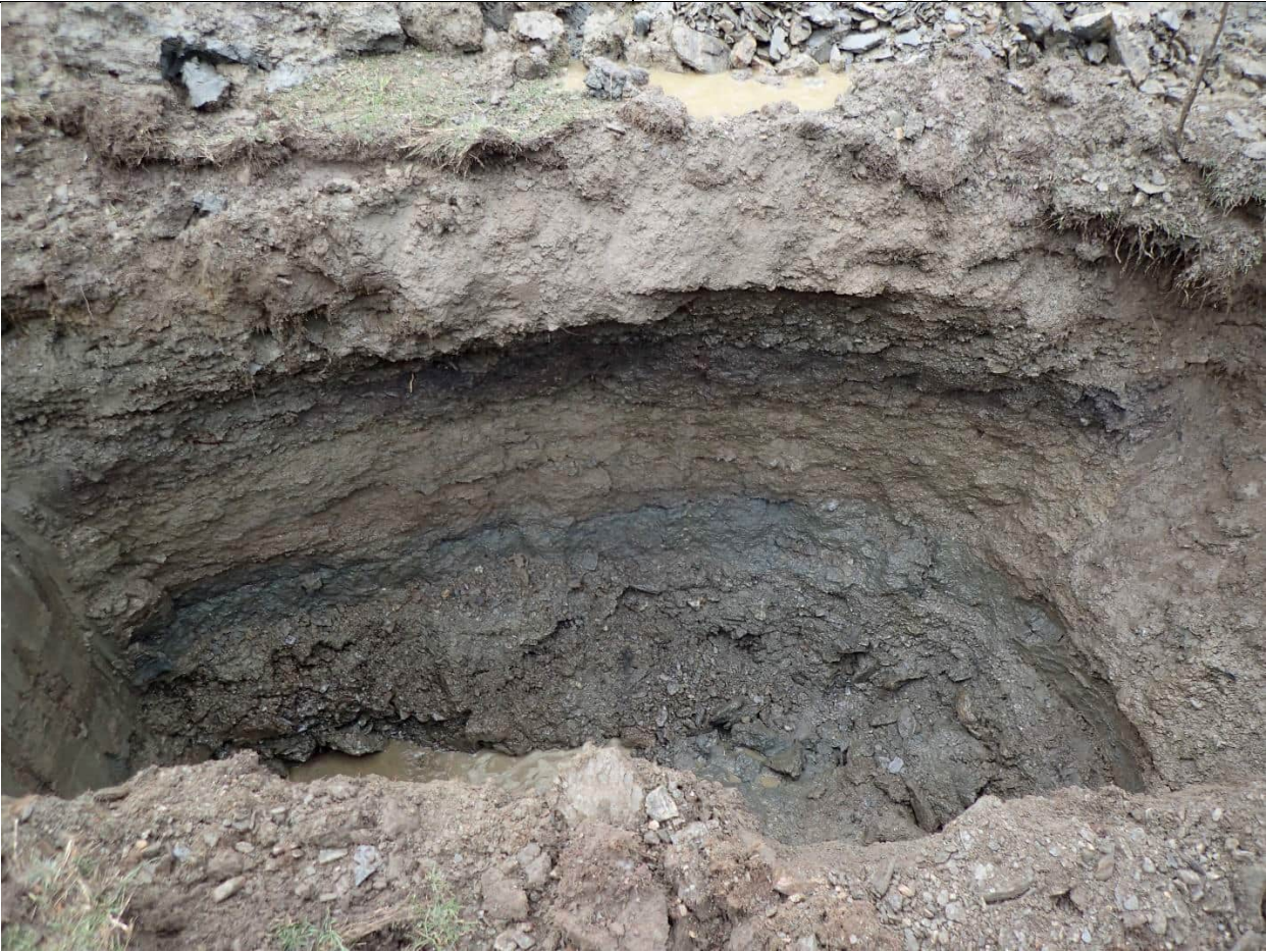
Testpit at completion. Max depth 3m
