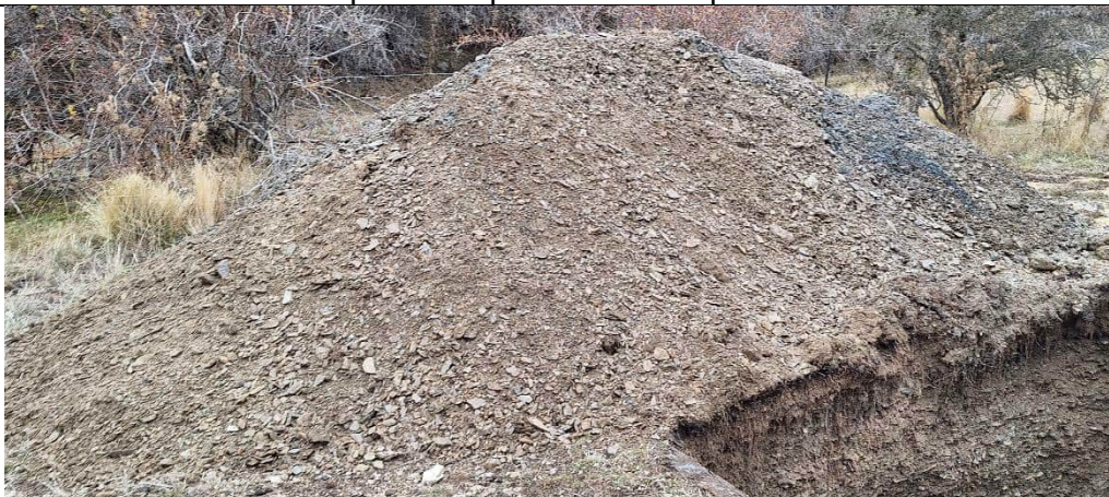
Spoil pile at end of excavation
