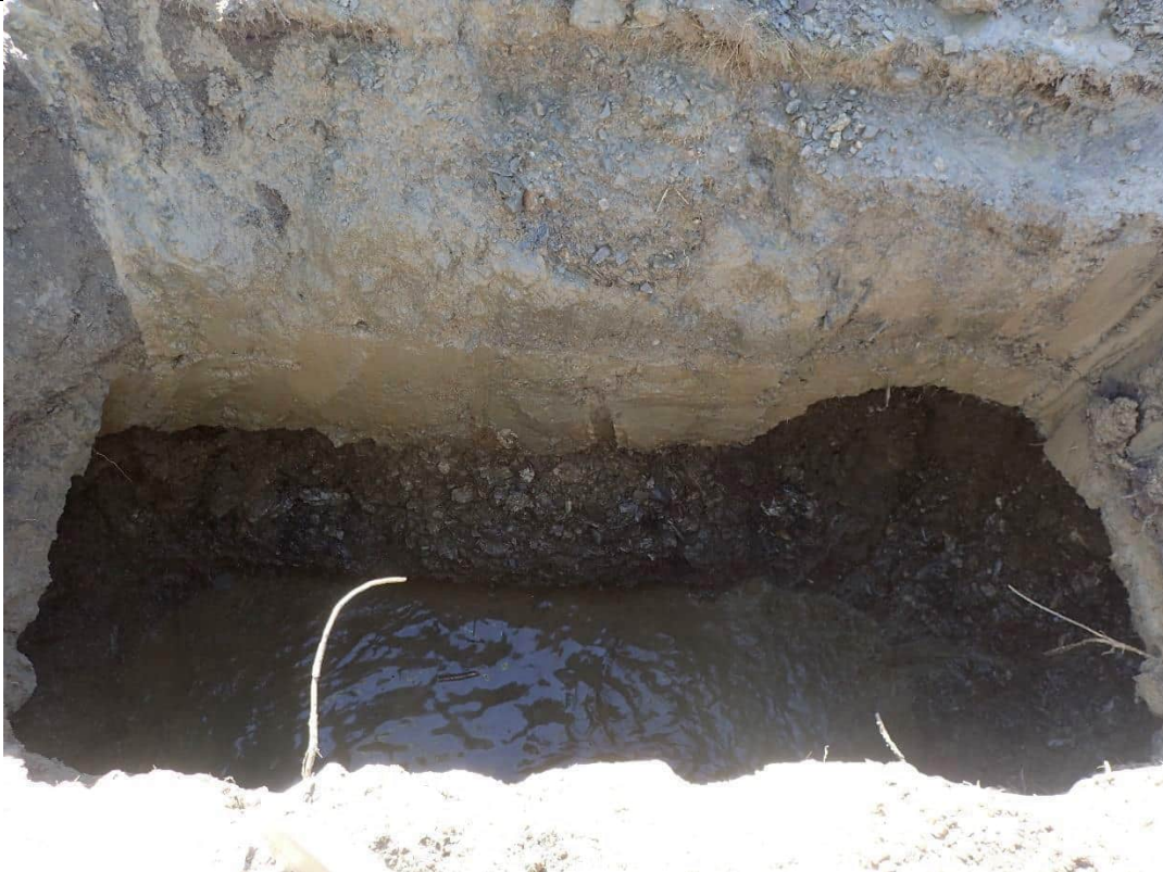
Testpit at completion. Max depth 6m
