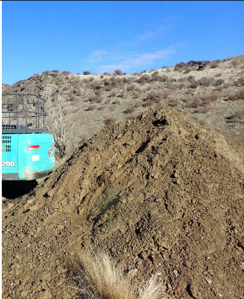
Spoil pile at end of excavation
