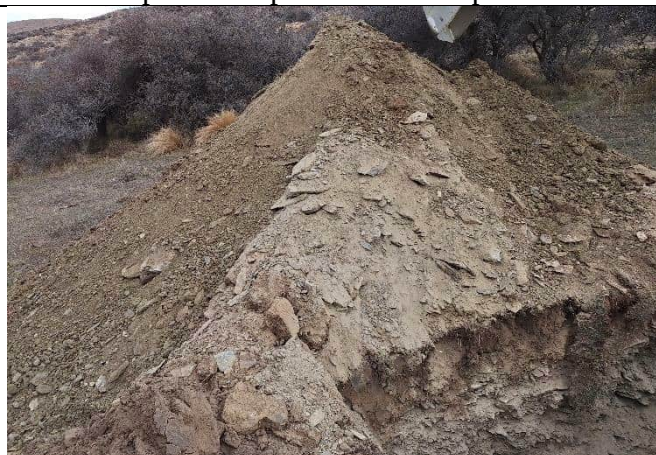
Spoil pile at end of excavation
