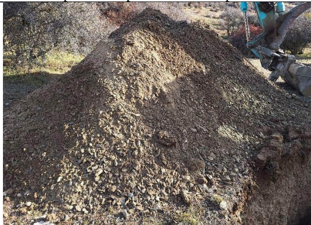
Spoil pile at end of excavation
