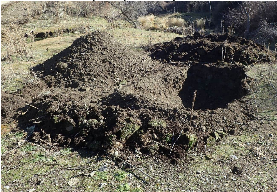
Spoil pile at end of excavation
