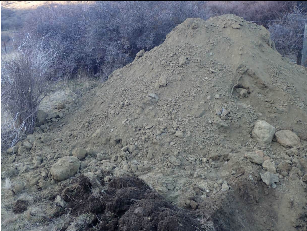
Spoil pile at end of excavation
