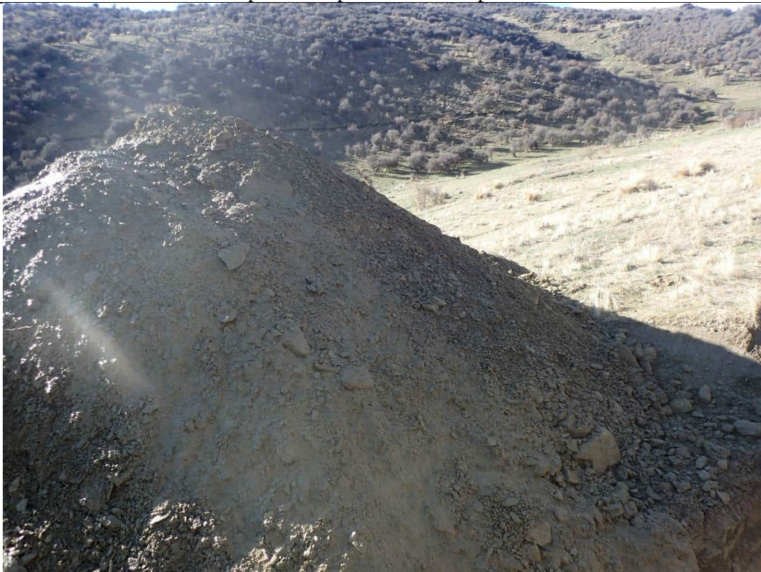
Spoil pile at end of excavation
