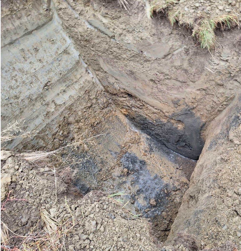
Testpit at completion. Max depth 2.6m
