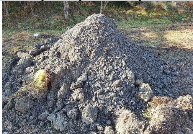
Spoil pile at end of excavation
