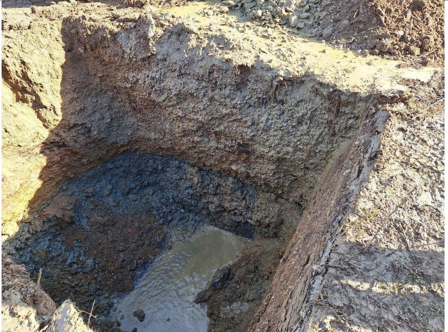
Testpit at completion. Max depth 2.7m
