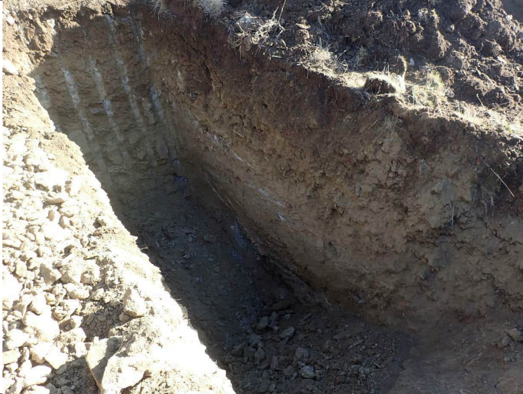
Testpit at completion. Max depth 2.5m
