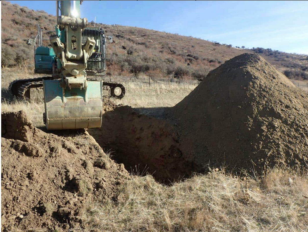
Spoil pile at end of excavation
