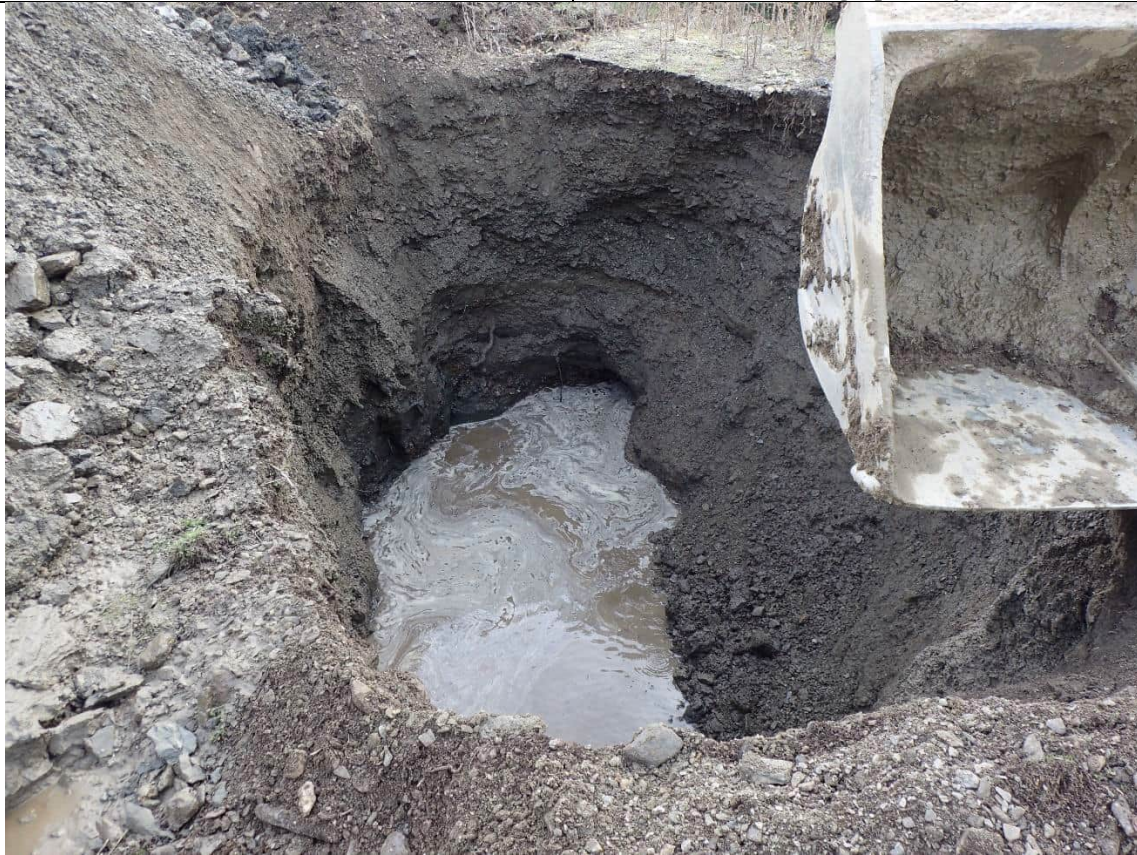
Testpit at completion. Max depth 5.5m
