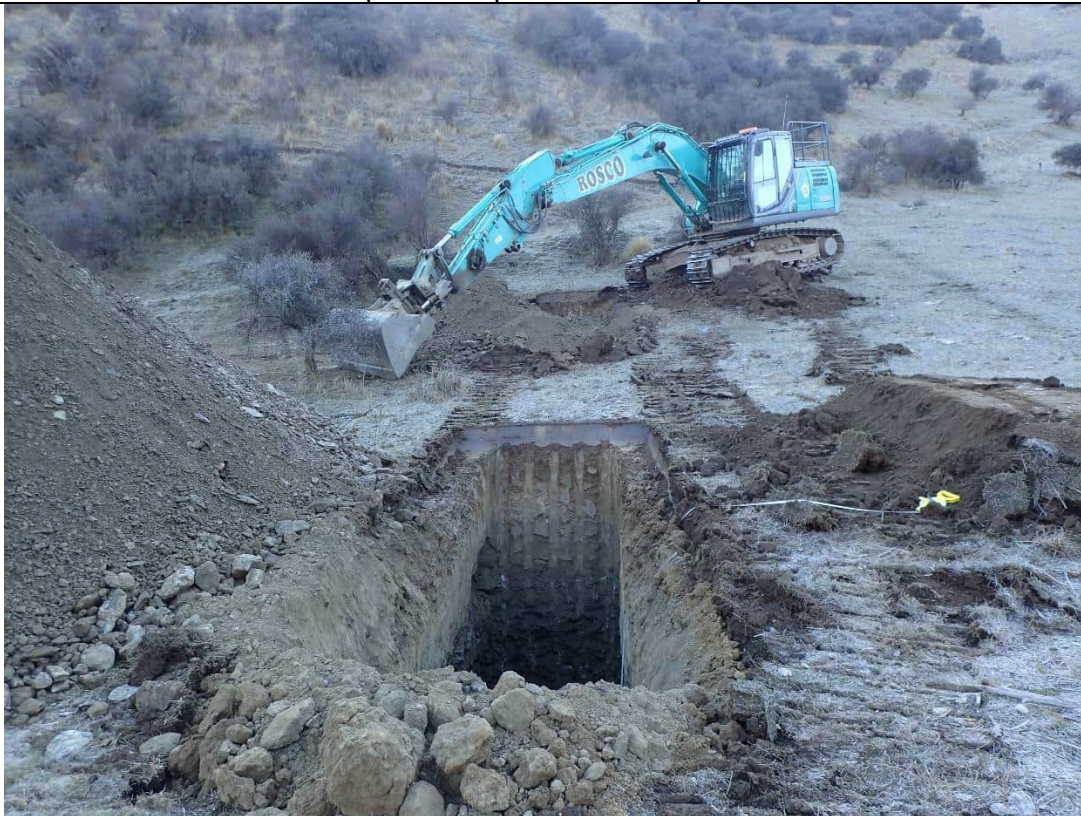
Spoil pile at end of excavation
