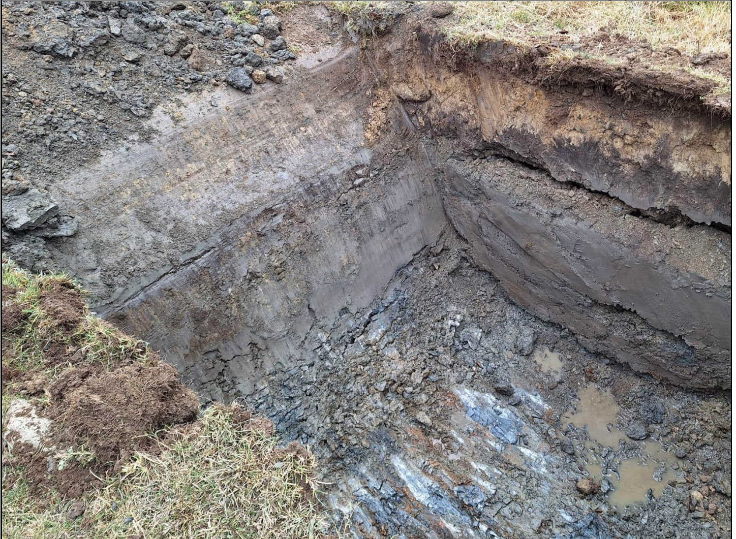
Testpit at completion. Max depth 1.9m
