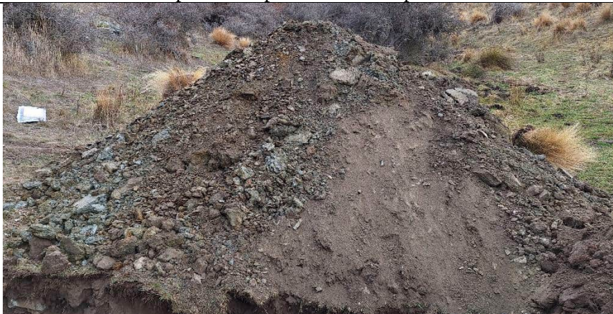
Spoil pile at end of excavation
