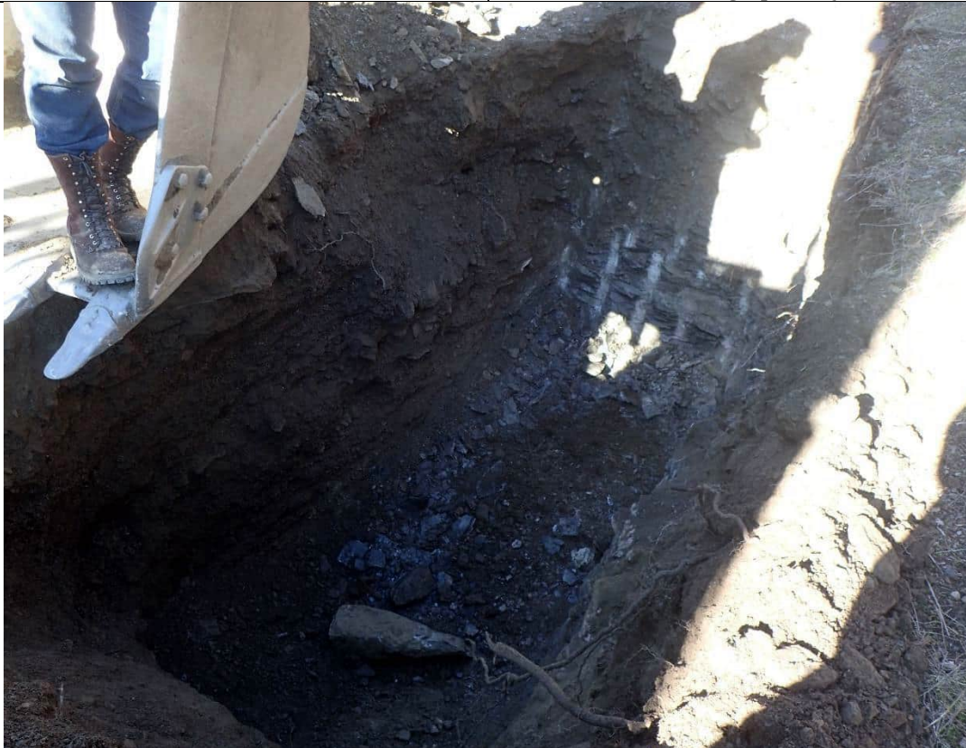
Testpit at completion. Max depth 2.5m
