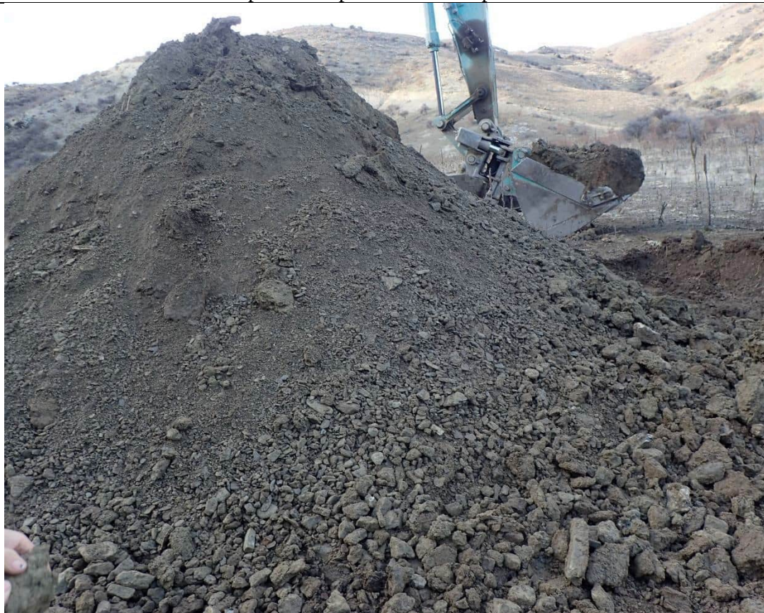
Spoil pile at end of excavation
