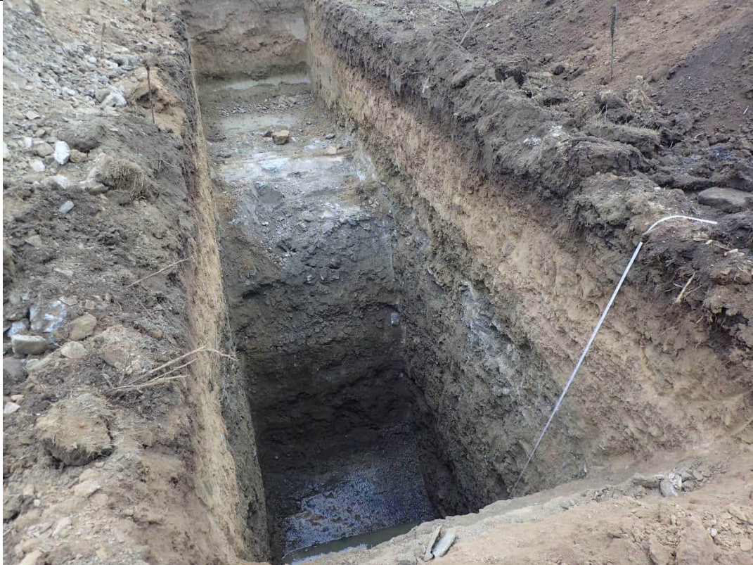
Testpit at completion. Max depth 6m
