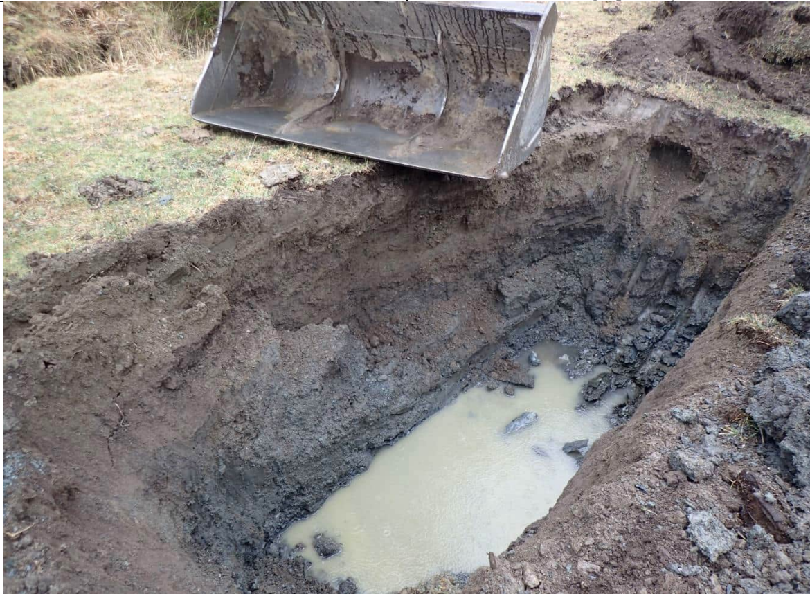
Testpit at completion. Max depth 2m
