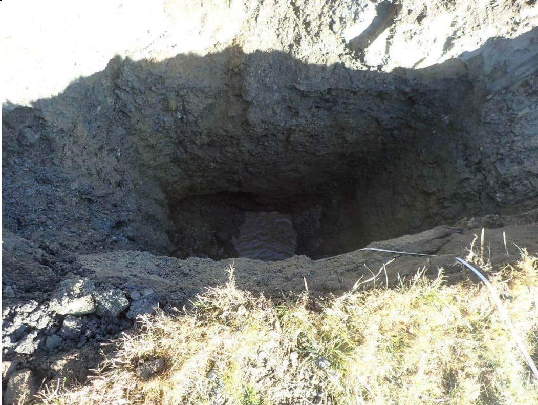
Testpit at completion. Max depth 5m
