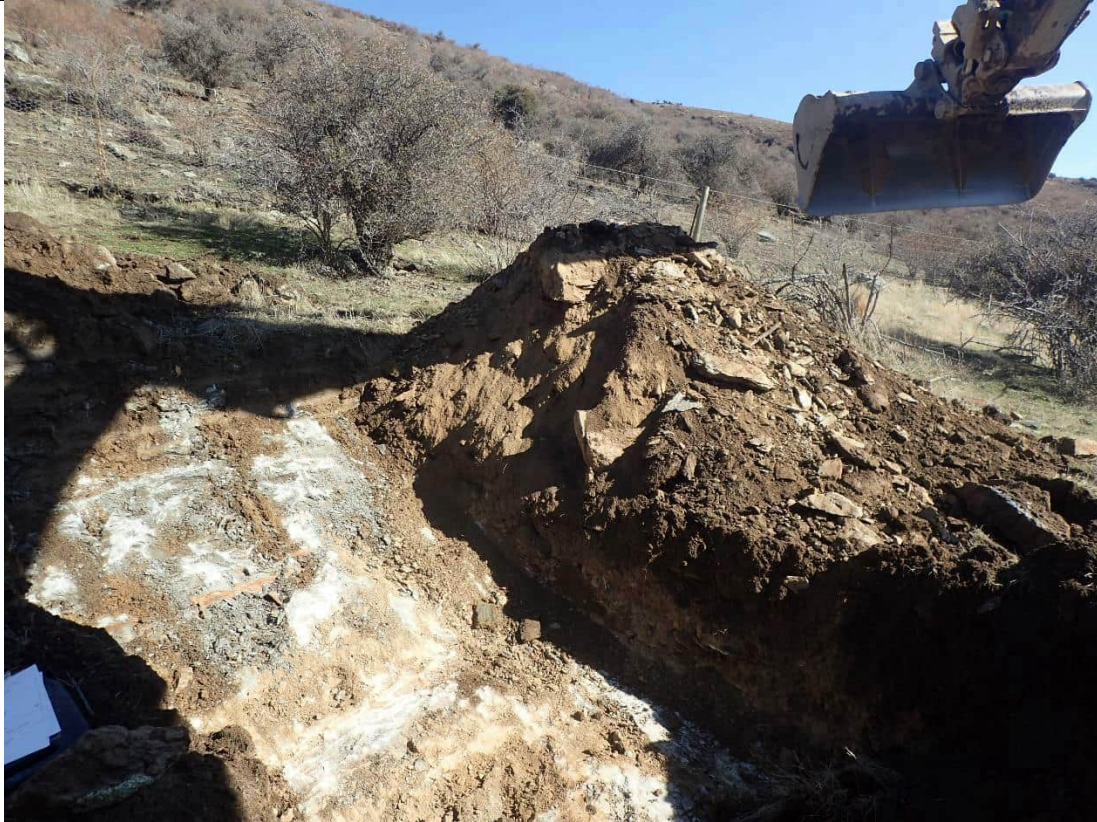
Spoil pile at end of excavation
