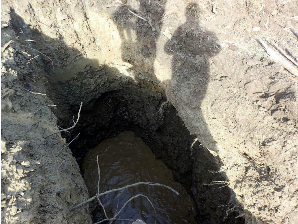
Testpit at completion. Max depth 4.5m
