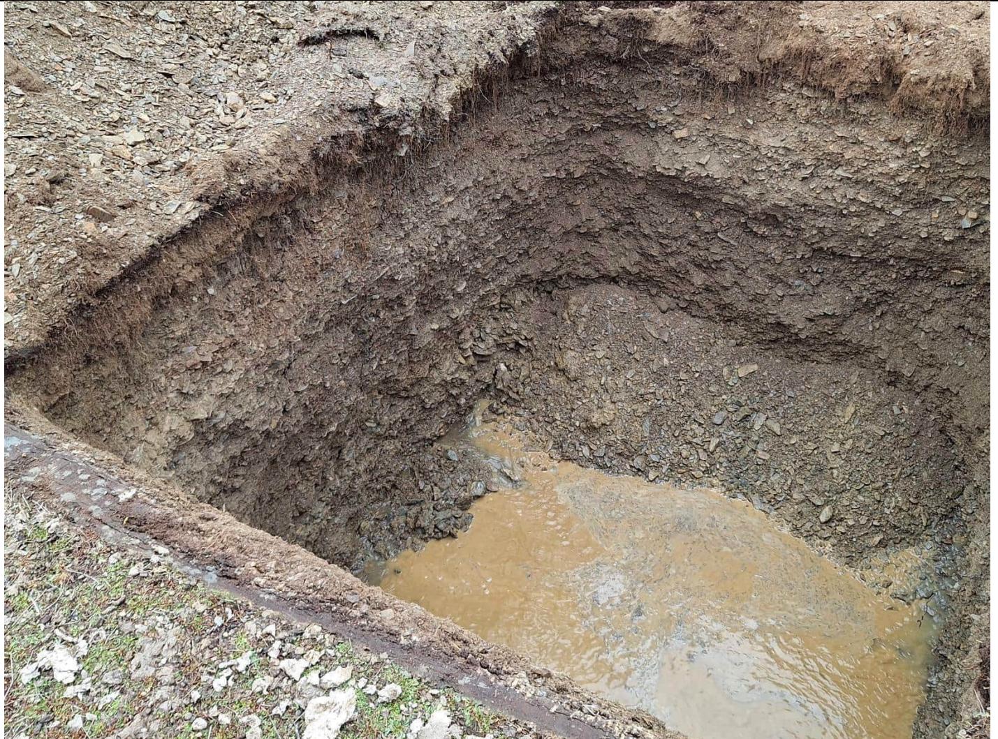
Testpit at completion. Max depth 2.4m
