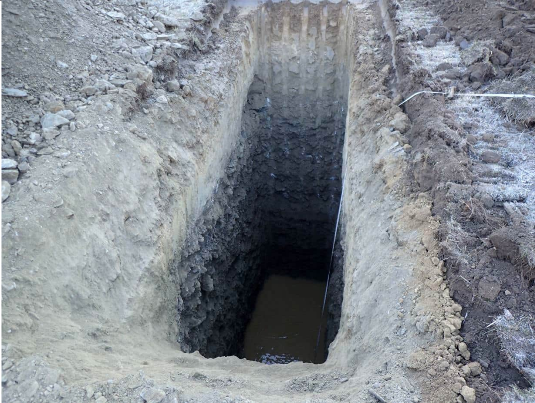
Testpit at completion. Max depth 7m
