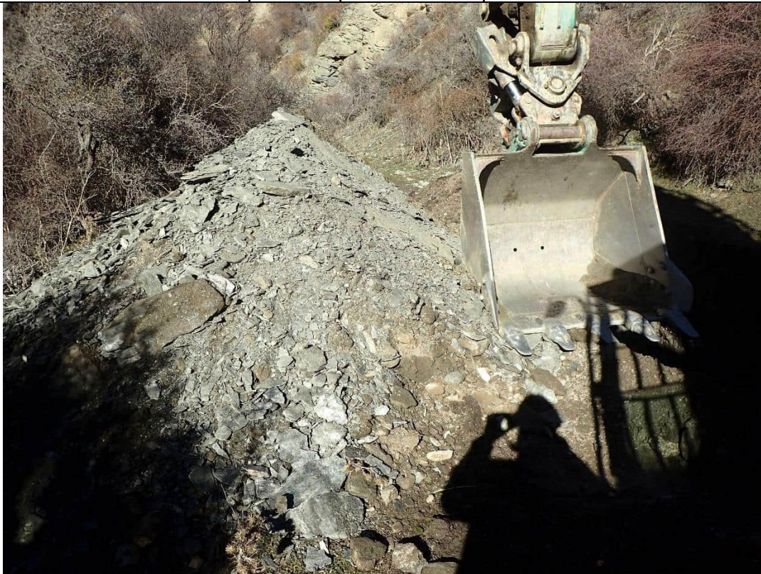
Spoil pile at end of excavation
