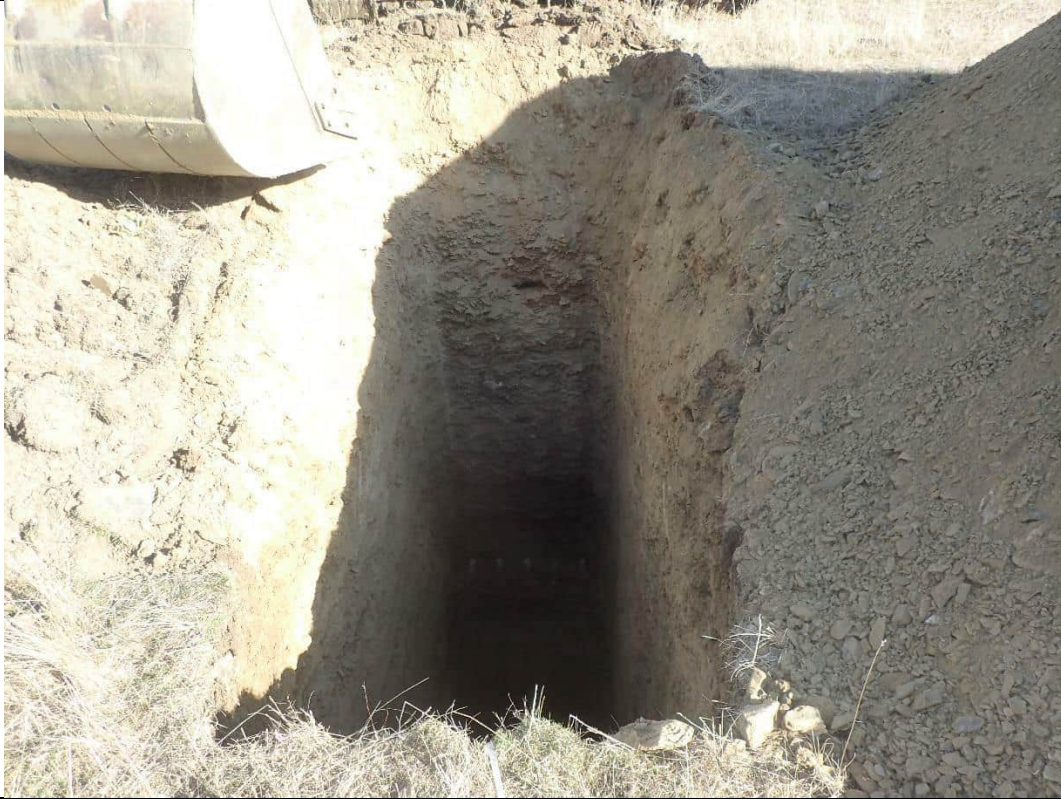
Testpit at completion. Max depth 6.5m
