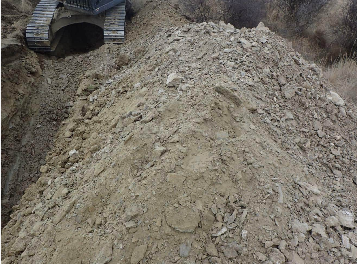
Spoil pile at end of excavation
