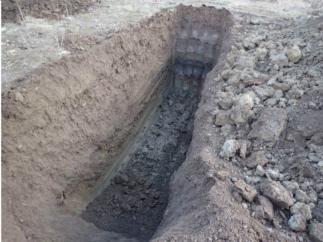
Testpit at completion. Max depth 4.5m
