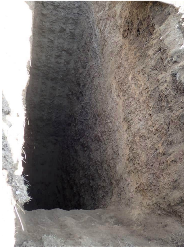
Testpit at completion. Max depth 7.5m
