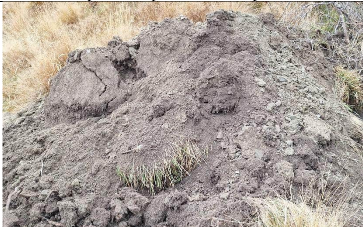
Spoil pile at end of excavation
