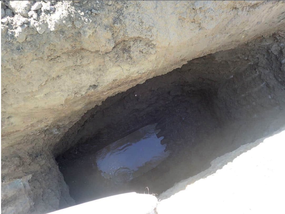
Testpit at completion. Max depth 6.5m
