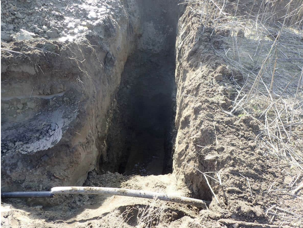
Testpit at completion. Max depth 6m
