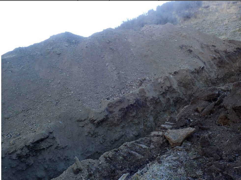
Spoil pile at end of excavation
