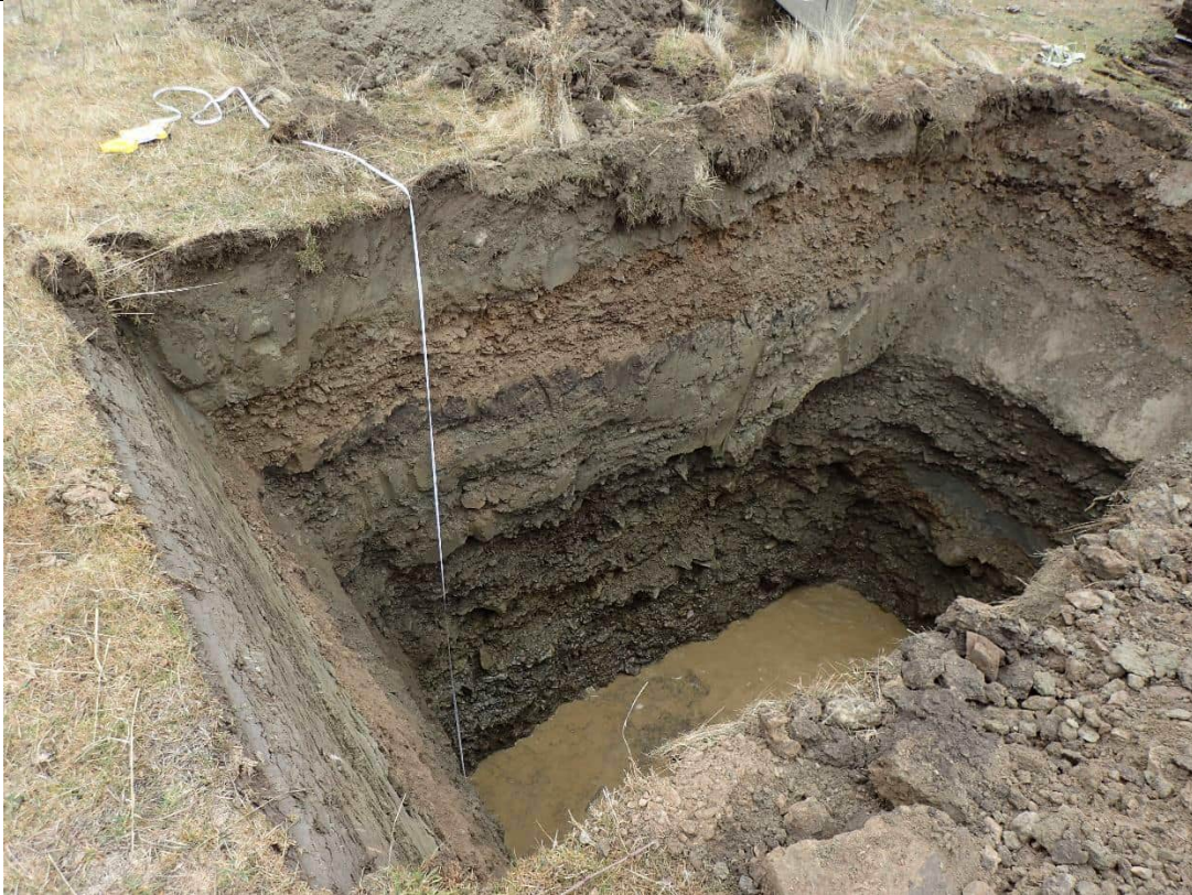
Testpit at completion. Max depth 6m
