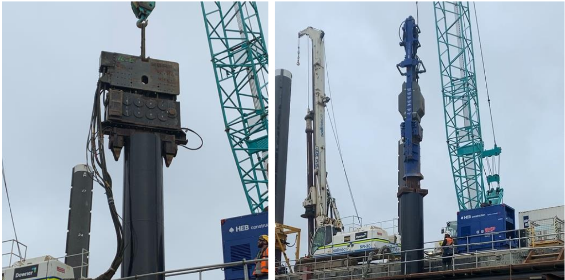
Figure 2: Vibro hammer (left) and impact hammer (right) source data used in our model
