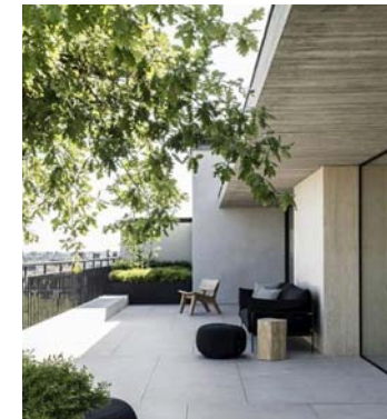
8 Landscaped roof terrace
