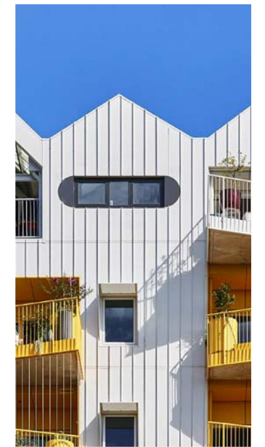
1 Metal cladding and roofing
