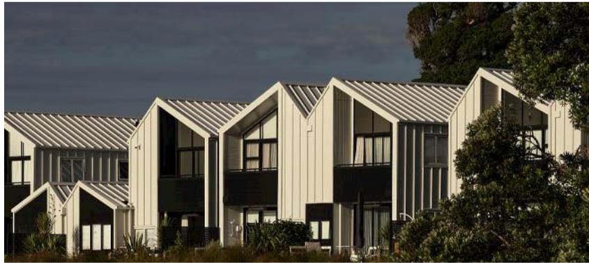
1 Metal cladding and roofing
