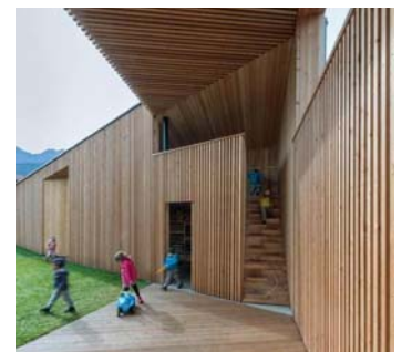
4 Stained timber cladding
