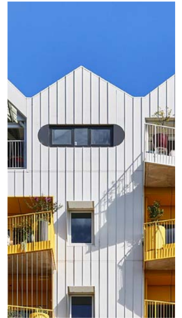
1 Metal cladding and roofing
