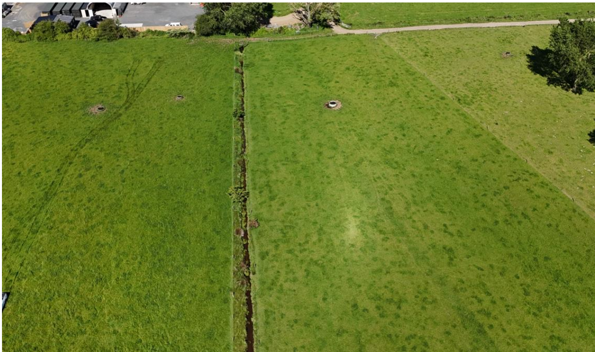
Figure 17. Location of a open field drain that coincides with georectified historic survey plans. Taken facing east with drone.
