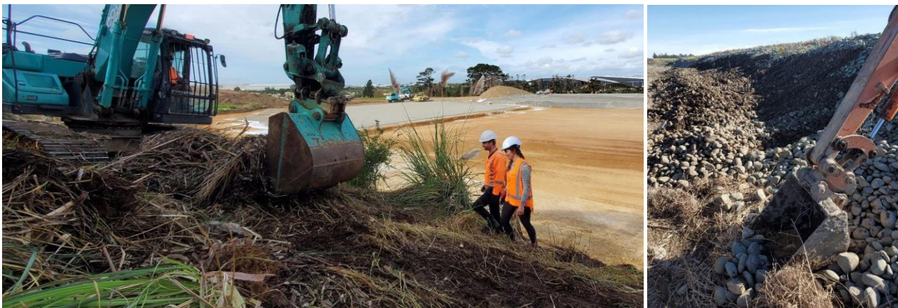
Figure 7. Machine-assisted lizard searches: in terrestrial vegetation (left) and cobble rock habitat (right).
