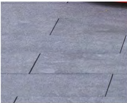
SU-107 Paving (Pedestals)
