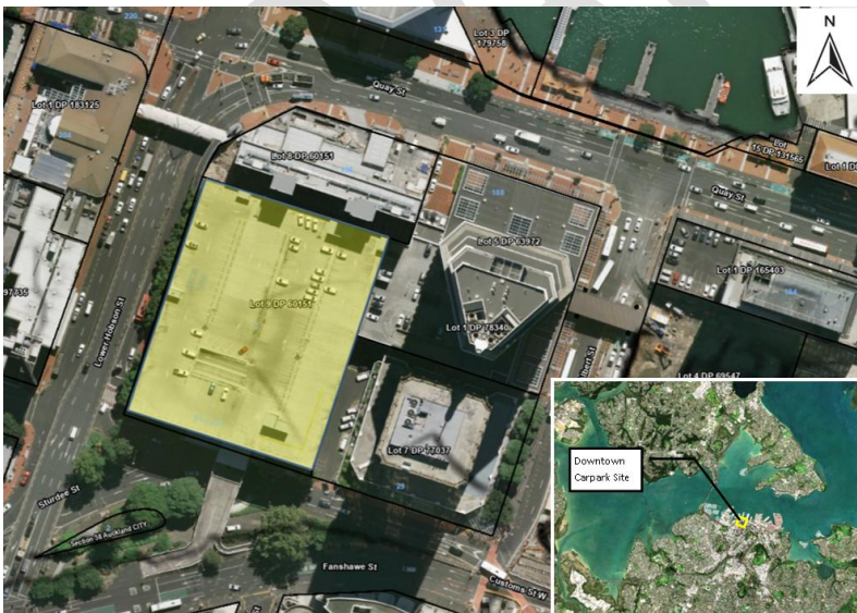
Figure 1.1: Downtown Carpark Development Site.
