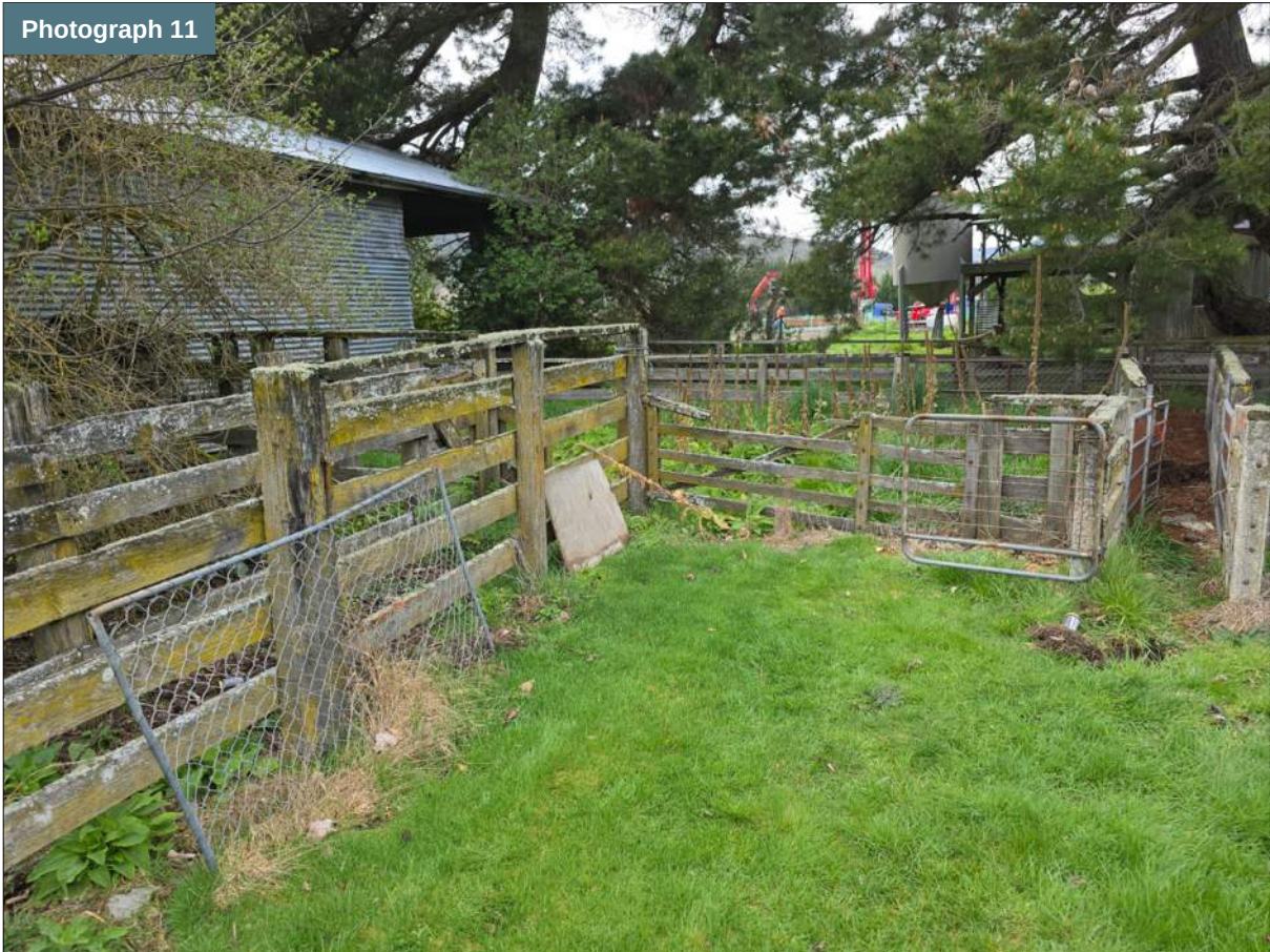
Holding pens/stock races south of the main livestock shed
