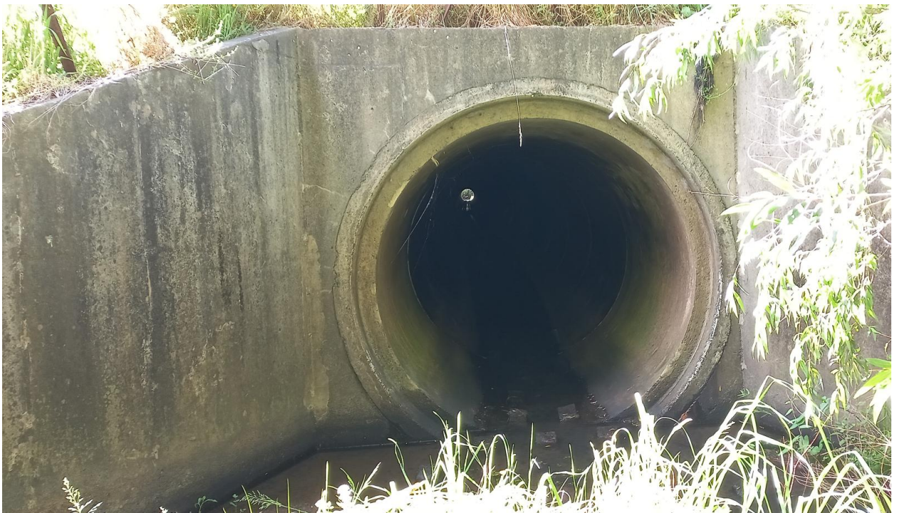
Figure 6 – Photo of culvert under State Highway 1
