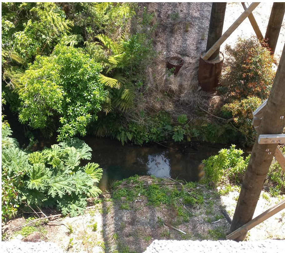
Figure 8 - Downstream bridge piles
