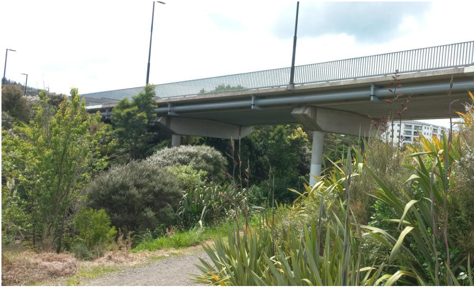
Figure 9 - Downstream bridge piles
