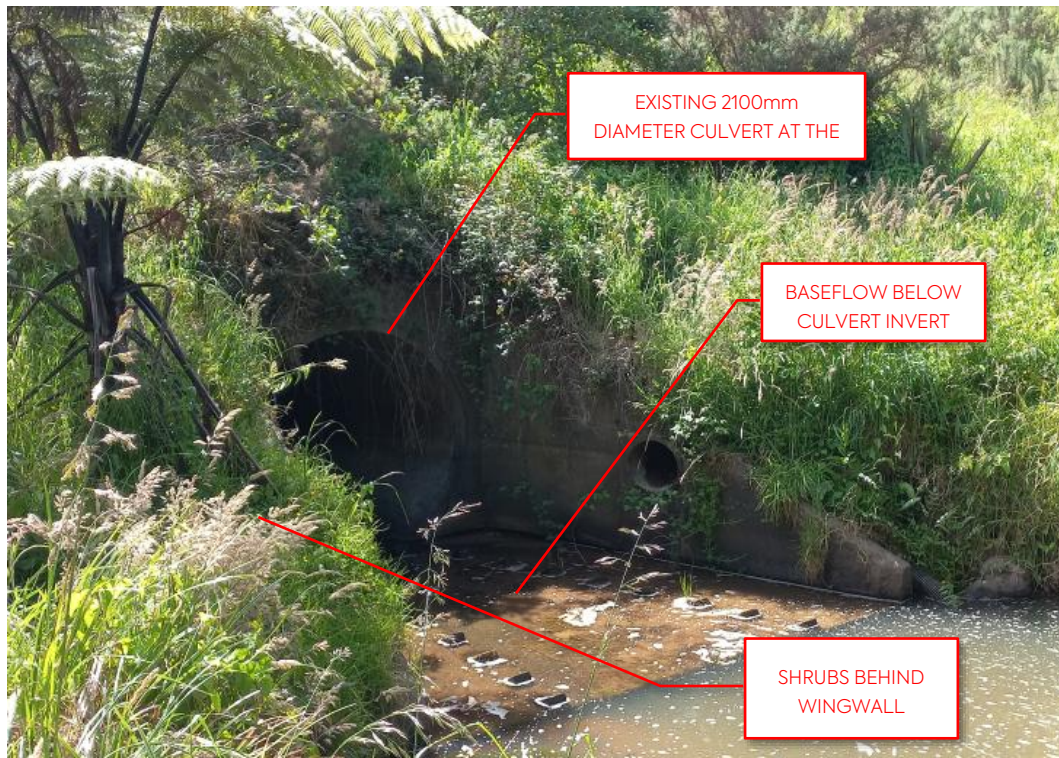
Figure 7 - Inlet of Culvert under State Highway 1
