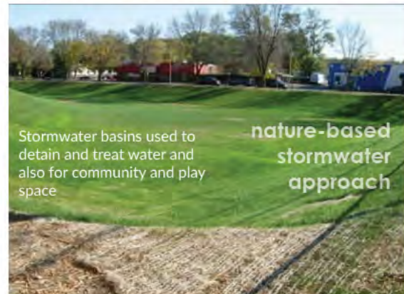
Stormwater basins used to detain and treat water and also for community and play space
