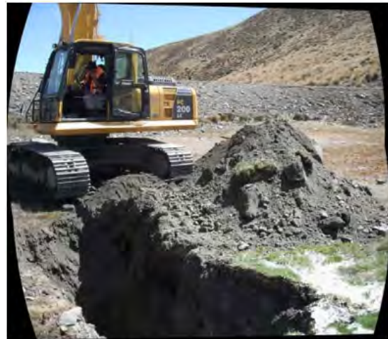
Figure 3-1 : Test pit excavation in pond 2.
