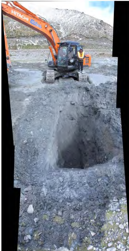
Figure 3-2 : Test pit profile showing dry graded colluvium in Pond 1
