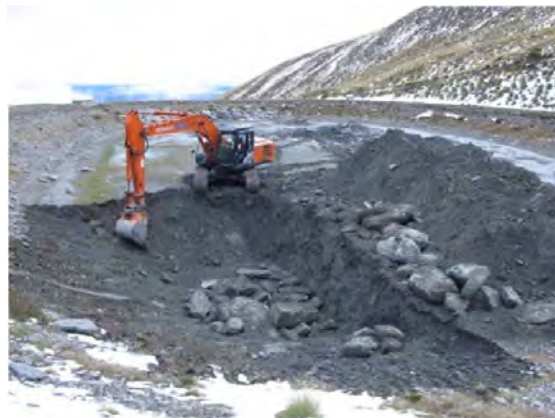
Figure 3-5 : Pond 1 during renovation operation
