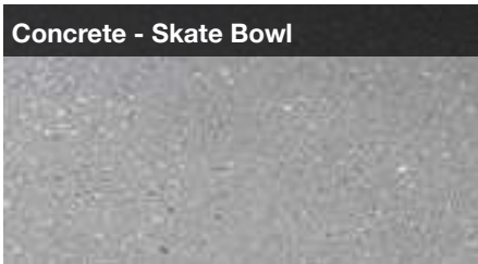
Honed concrete suitable for a skating
