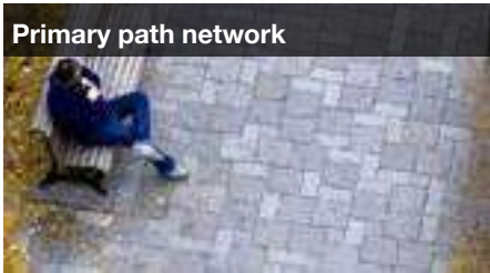
Concrete pavers for primary circulation and entries.
