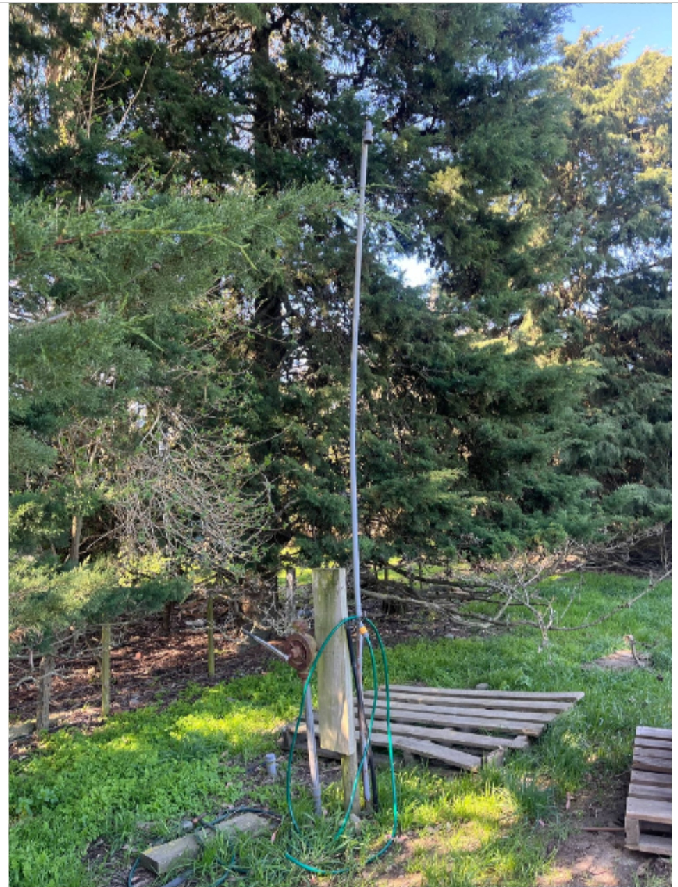
Fuel dispenser by area of presumed below ground storage tank
