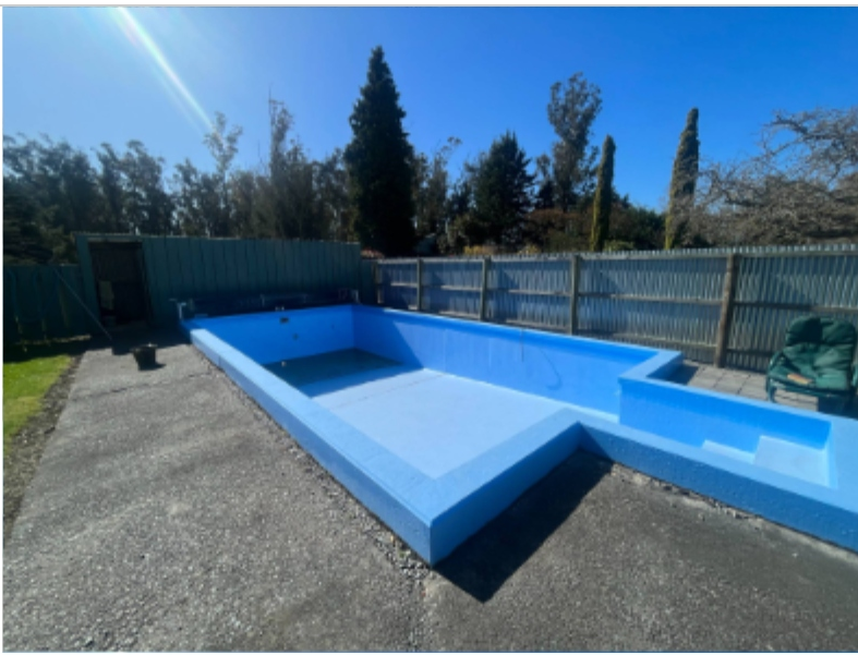
Pool area to west of dwelling
