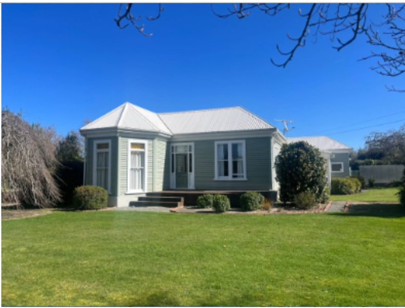
Onsite dwelling looking west from lawn area
