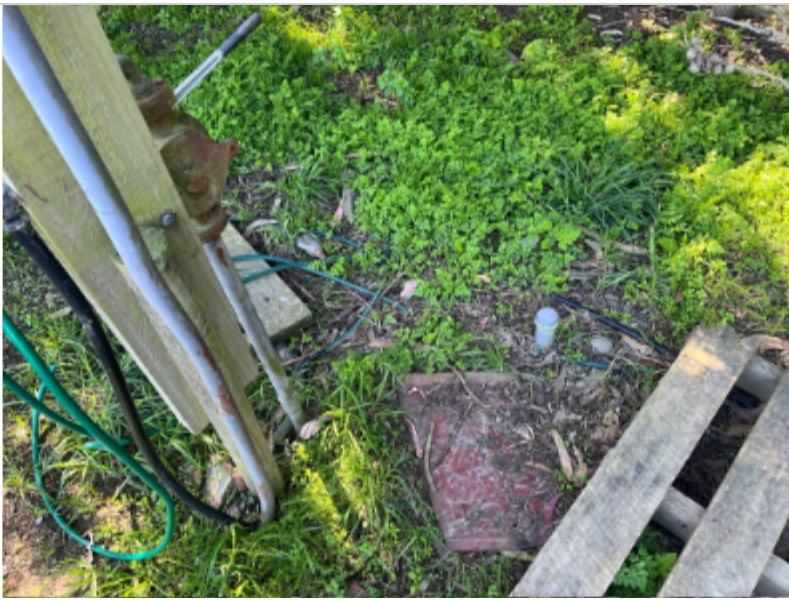
Visible vent by area of presumed underground storage tank
