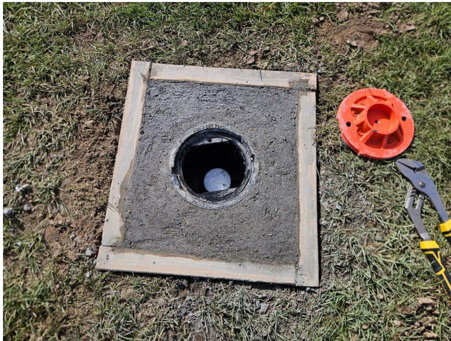
Photo 8: KP02 Flush mounted to by 09-02-2026. Subsequently lowered to finish a few cm below ground level
