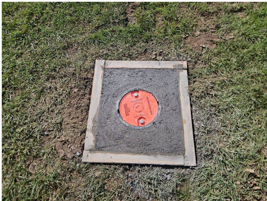
Photo 8: KP02 Flush mounted to by 09-02-2026. Subsequently lowered to finish a few cm below ground level
