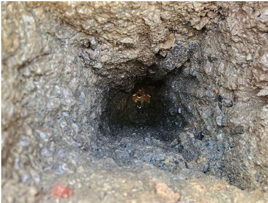
Photo 4:KP02 End of hydrovac 1.5 m depth 09-02-2026
