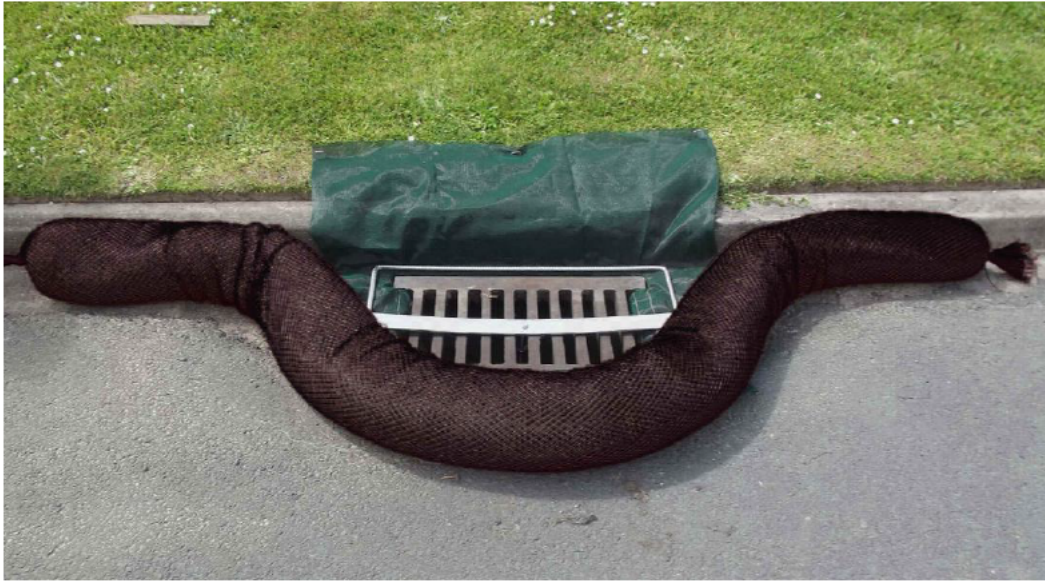
Figure 12: SW sump catch pit protection example with filter bag & silt sock
