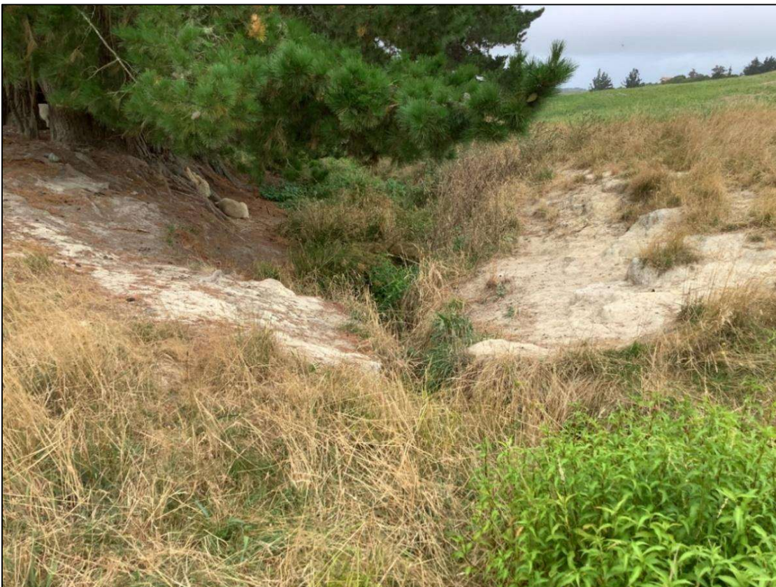
Plate 7: The incised upper reaches of Stream R5 flow intermittently and were predominantly dry at the time of the site visits in summer (February 2022). Previous and current land uses have resulted in the loss of riparian vegetation and exacerbated severe erosion of stream banks.
