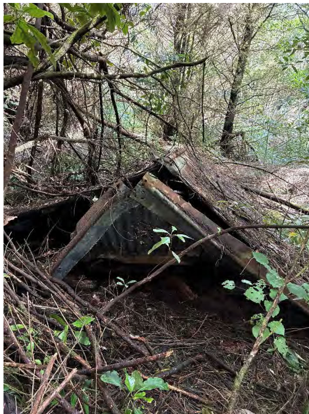
Photograph 2: Example of roof structure.
