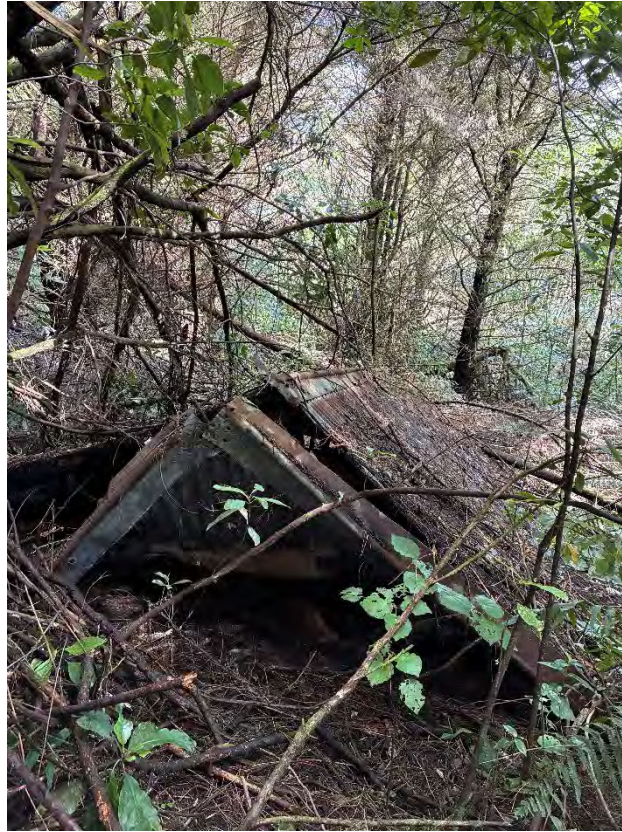
Photograph 9: Roof structure at former dwelling (SS05).
