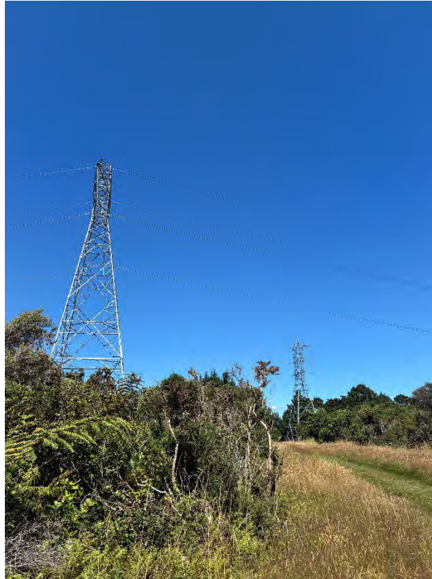
Photograph 1: View of onsite pylons, looking north.
