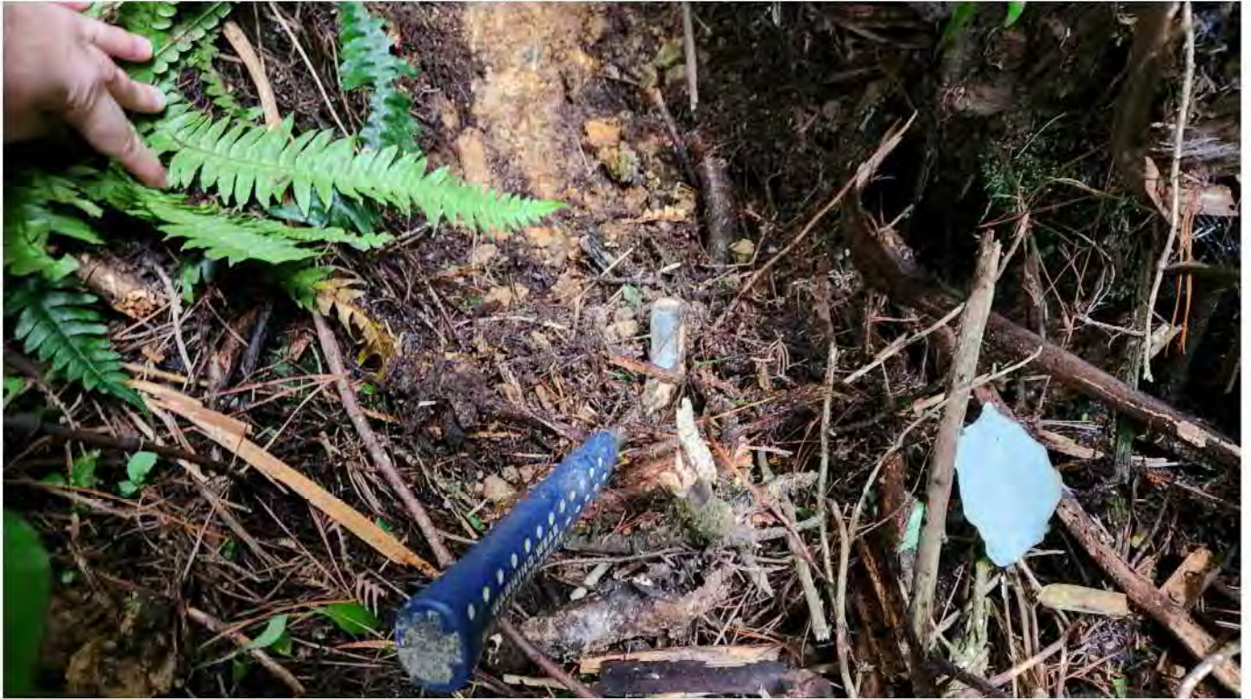
Photograph 1: Completely weathered Greywacke in watercourse, start of groundwater seepage at location Bx01 [eastern sidling gully]. Downstream gully remains dry.
