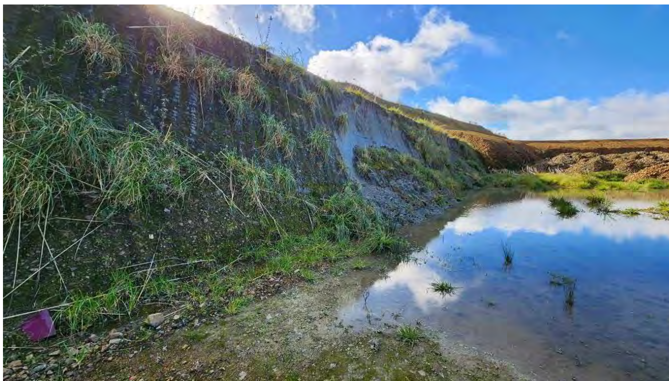
BQ14: Lowermost batter in pond fines illustrating localised failure and contact with backfill.
