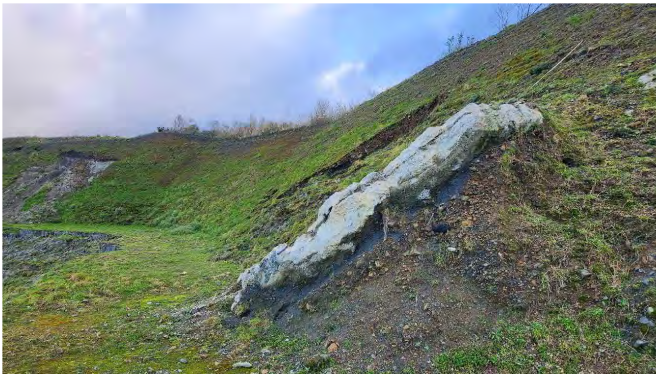
BQ03: Historic backfill overlain by waste concrete and process fines.
