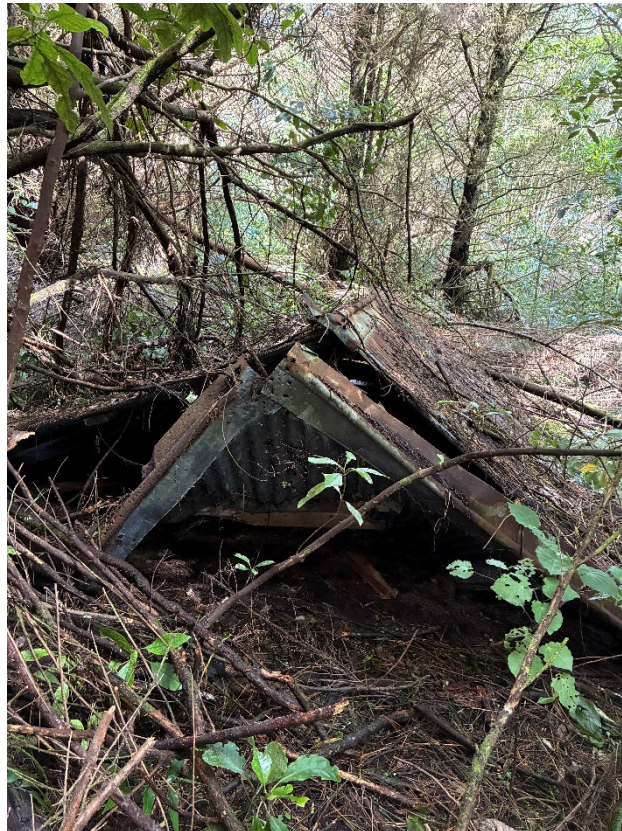
Photograph 2: Example of roof structure.
