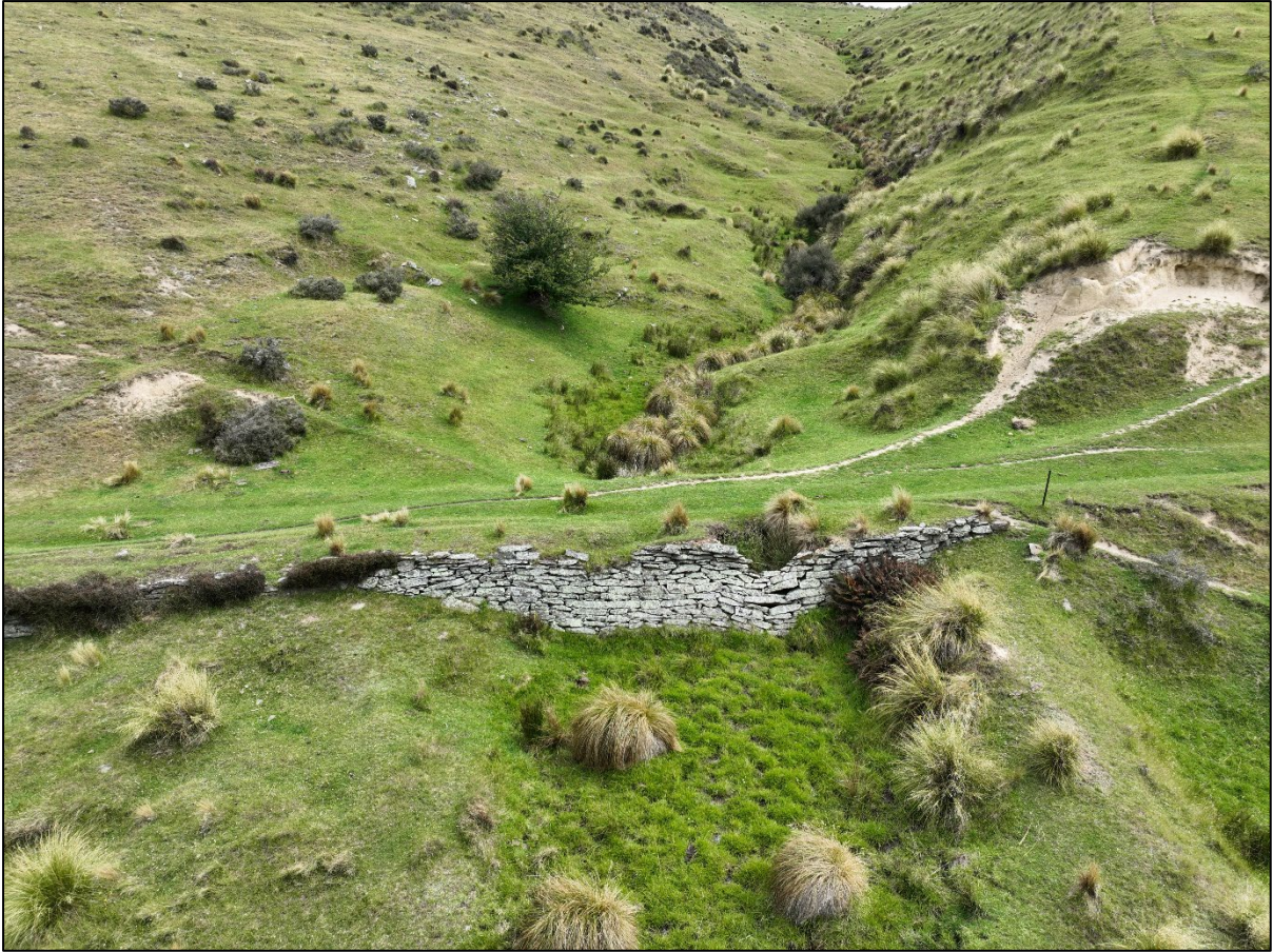
Figure 111. Major revetment, looking south-west.
