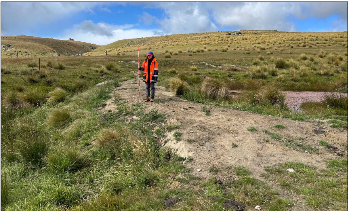
Figure 163. Dam, looking south-east.
