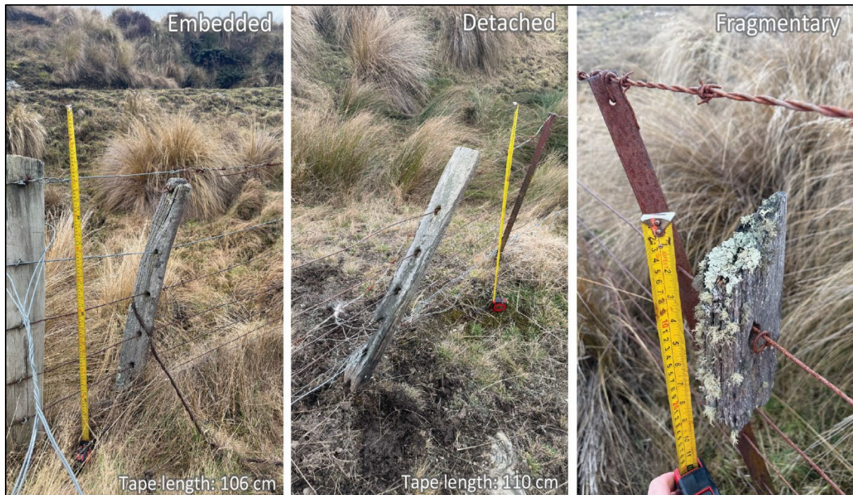
Figure 173. Different states of fence posts along fence line I42/257.
