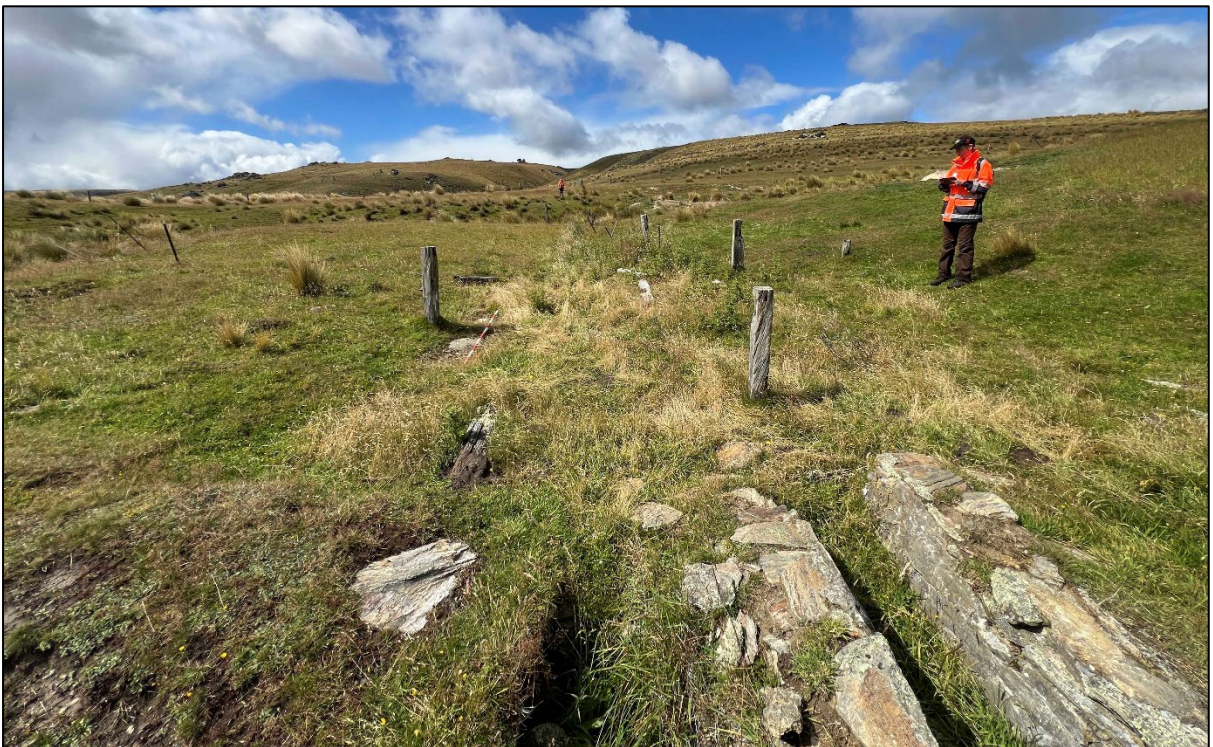
Figure 165. Remnant fenceposts from yards at dip inlet, looking south-east.
