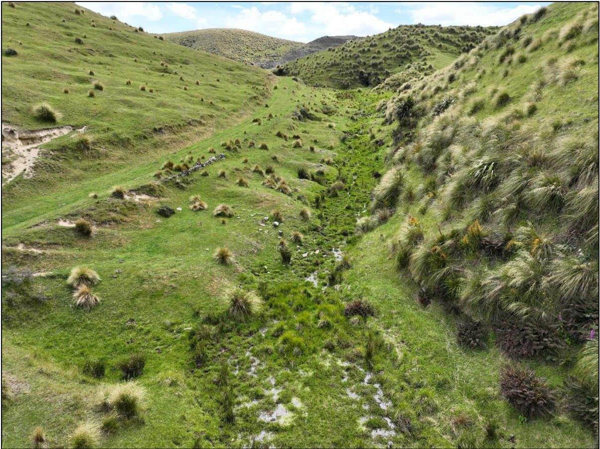
Figure 109. Revetment along track, looking north-west.
