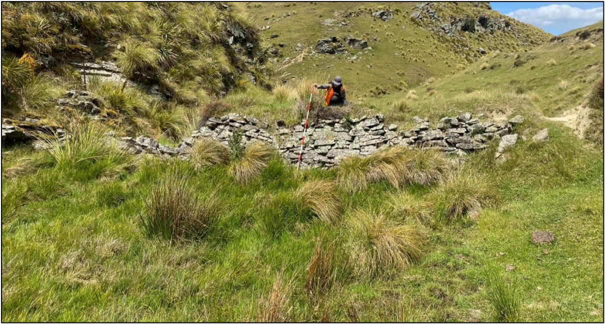
Figure 79. Dam (D), looking south-east. Breach noted by Petchey on the left.
