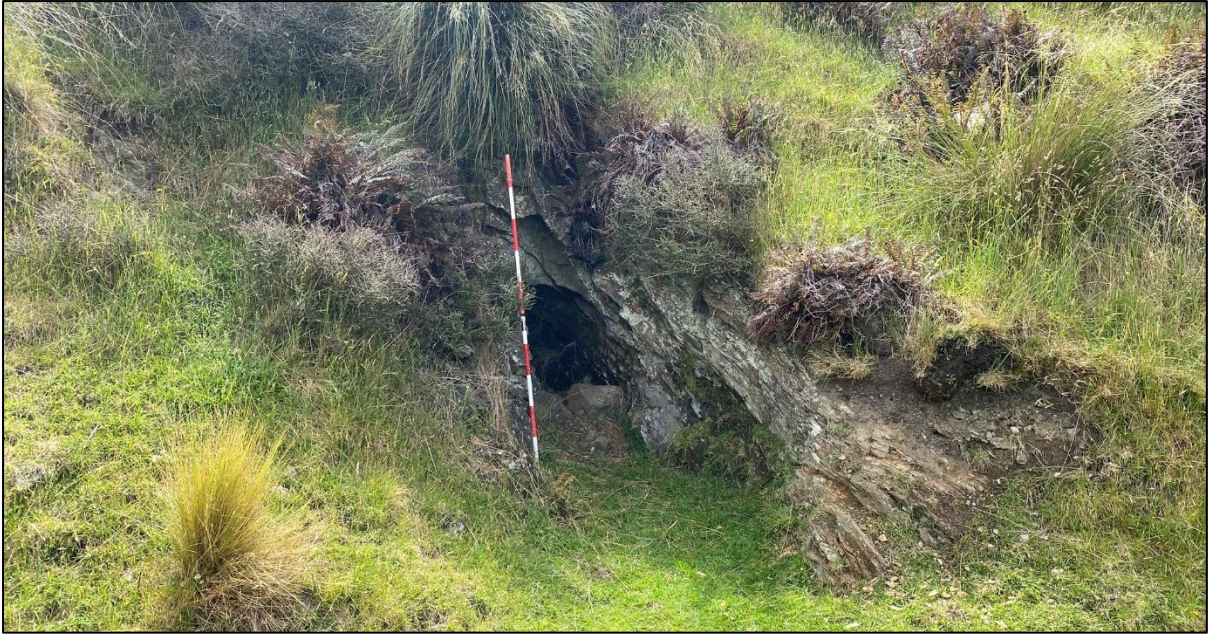
Figure 67. Adit feature (AD) adjacent to tramway, looking north-west.
