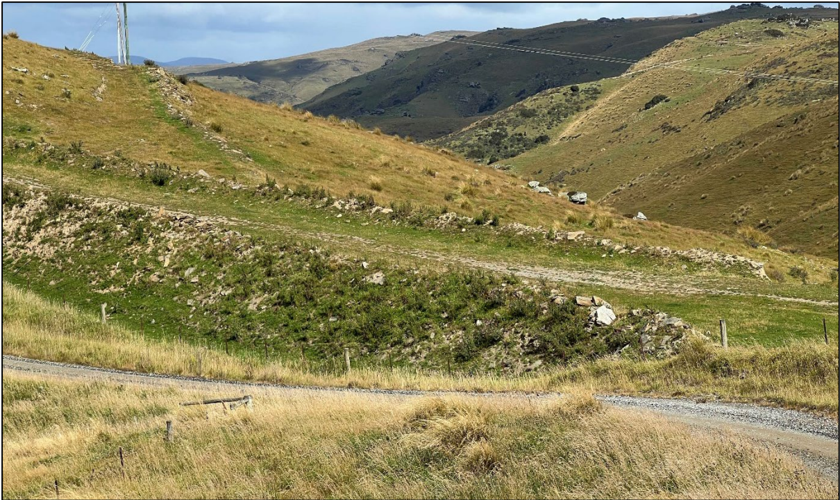
Figure 133. Example of the existing haul road formation, with Golden Bar Road in the foreground.
