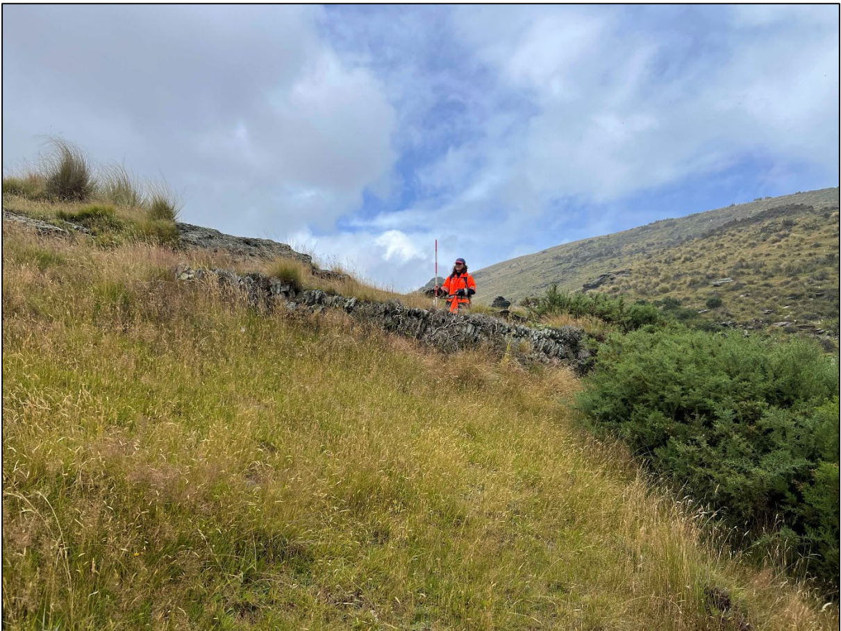
Figure 156. Stone revetment supporting the Ounce Battery water race (G) around the spur, looking south-east.
