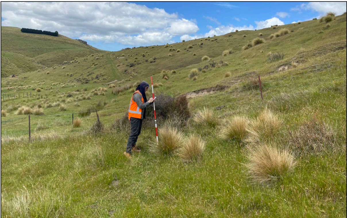
Figure 117. Looking along water race (WR), looking south-east.
