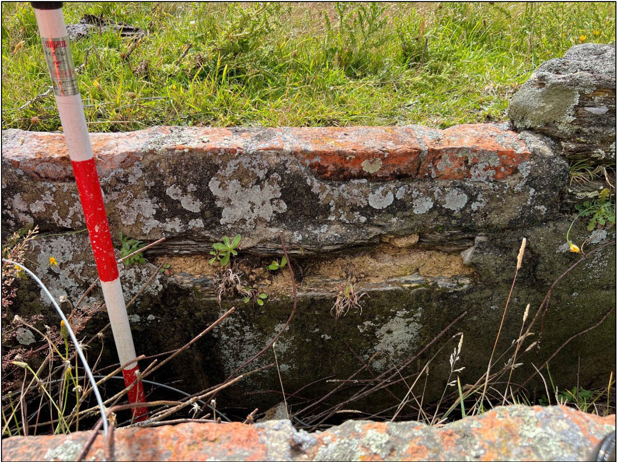
Figure 162. Detail of sheep dip showing mortared stone construction and brick top course.
