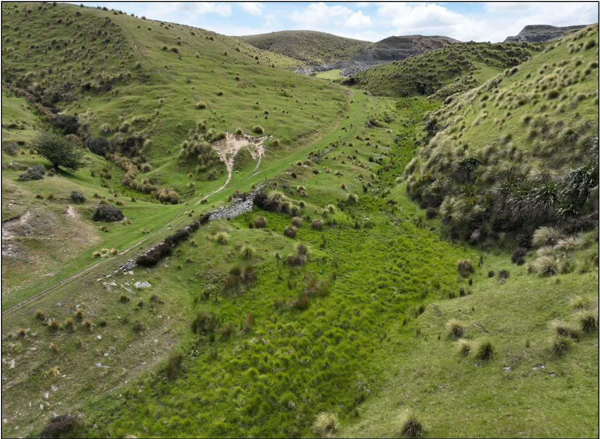
Figure 112. Showing the major revetment along the track in relation to the creek, looking north-west.
