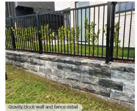
Gravity block wall and fence detail Image Stonefields development site
