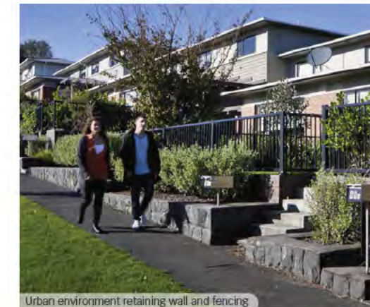
Urban environment retaining wall and fencing Image Internet source
