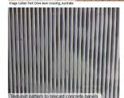
Textured pattern to precast concrete panels Image IC Darling Harbour, Australia
