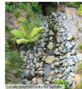
Locally sourced rocks for outfalls Image Ki uta ki tai, shared path Meadowbank
