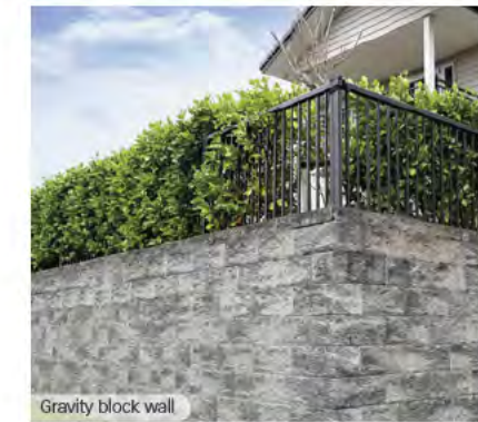
Gravity block wall Image Firth wall
