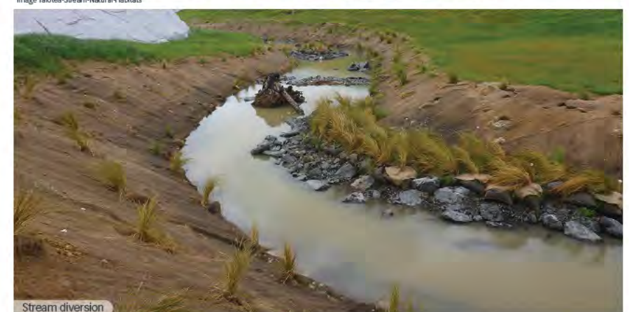
Stream diversion Image Stream diversion, Huntly bypass
