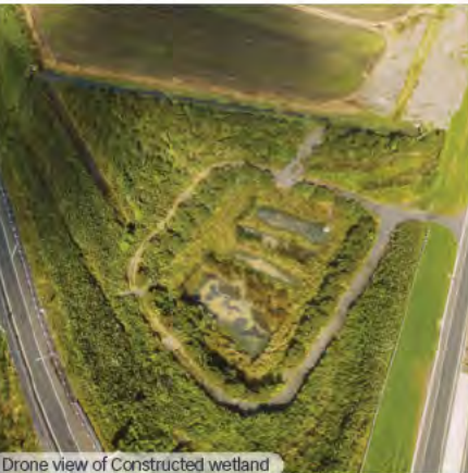
Drone view of Constructed wetland Image Waikato-Expressway-Infrastructure-Planting-Natural-Habitats
