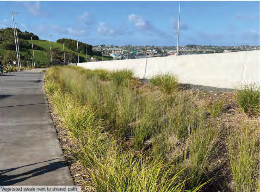
Vegetated swale next to shared path Image Northern corridor Auckland
