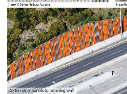
Corten steel panels to retaining wall Image Transmission Gully, Wellington
