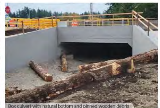
Box culvert with natural bottom and pinned wooden debris Image Internet source
