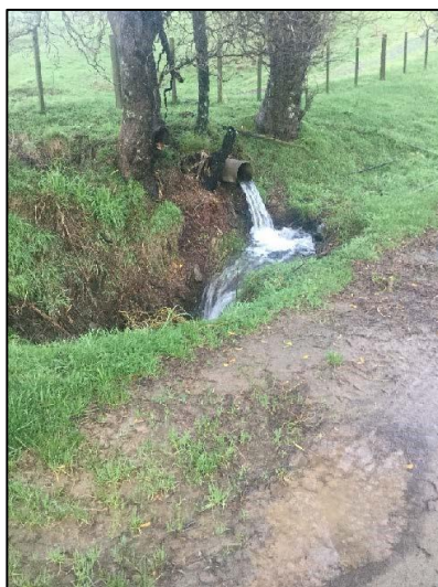
Figure 3-53: Perched Culvert on Tributary 2
