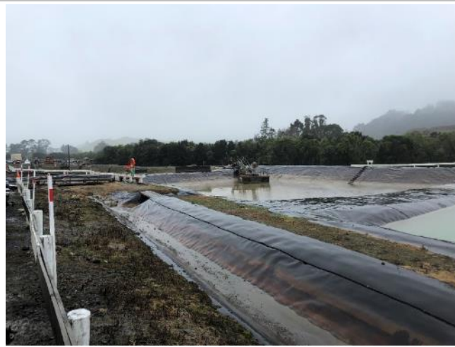
Photograph 12. Collection ponds for water from underground mine and site stormwater.
