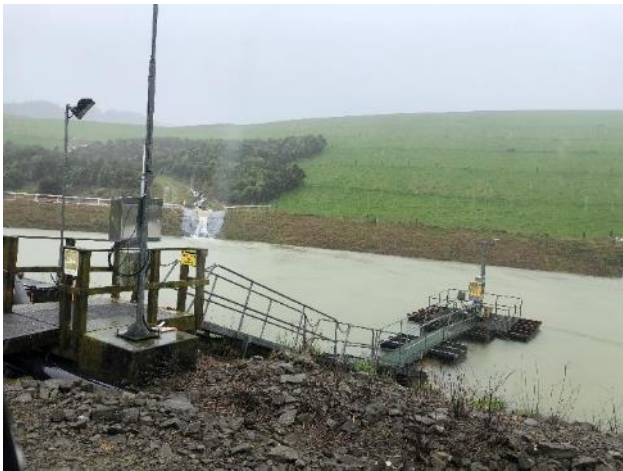
Photograph 29. Water spilling off TSF2 embankment to the collection pond.
