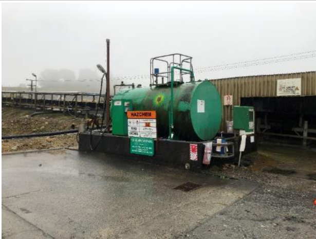
Photograph 7. Bunded diesel tank next to the conveyor.
