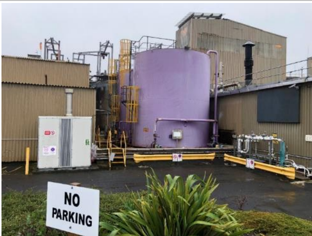
Photograph 3. Liquid cyanide tanks (purple).
