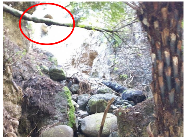
Photo 29. Perched culvert (red circle)
