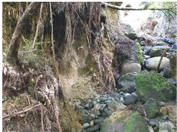
Photo 25. Scoured banks within Stream 7
