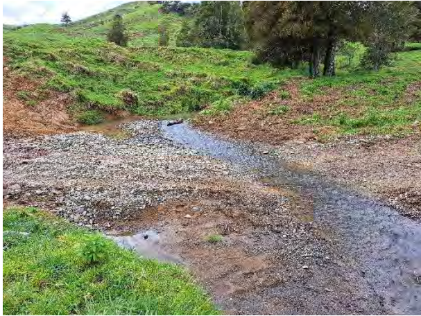
Photo 25. Low profile ford crossing in the centre of Tributary 1.
